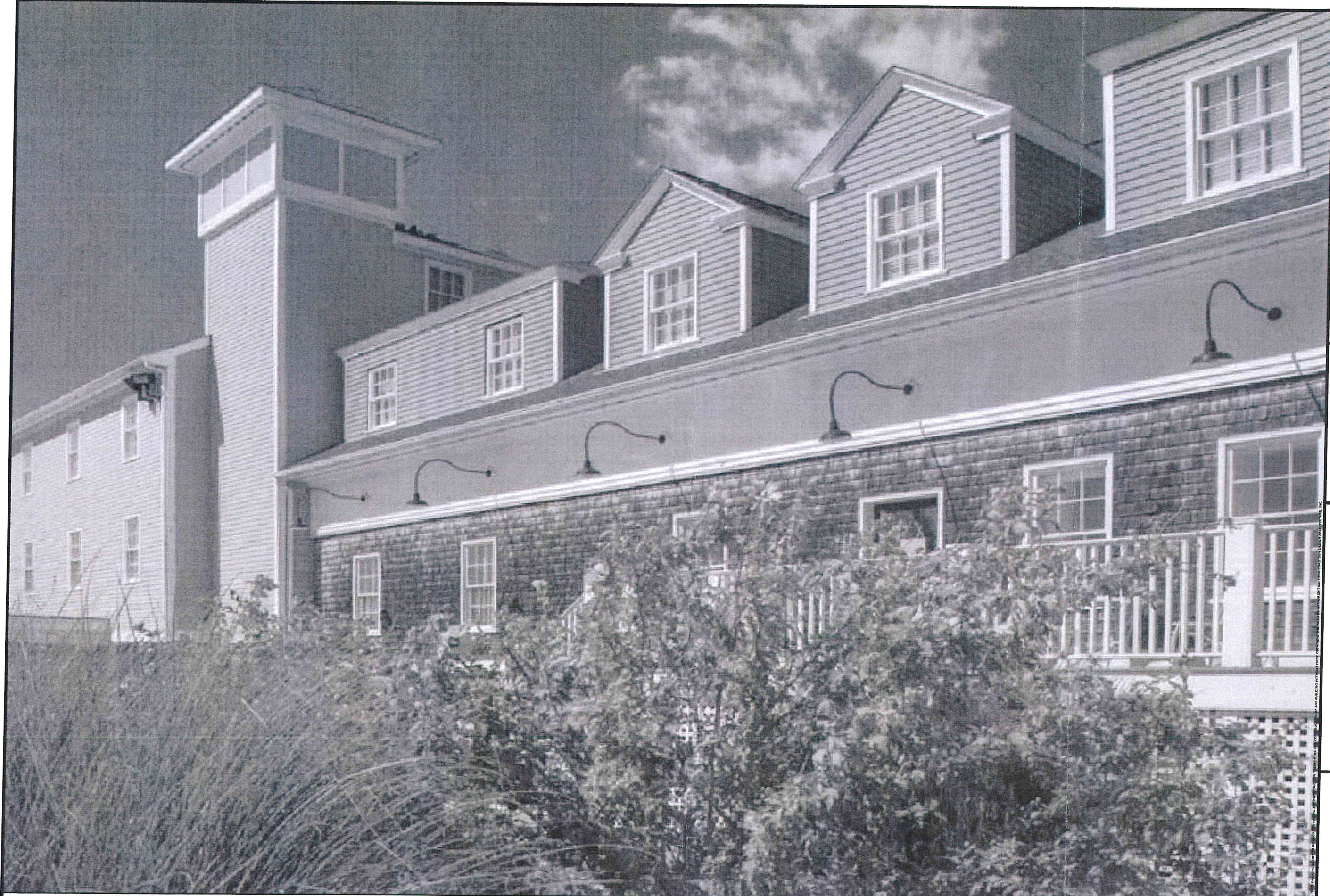
① EXTERIOR PHOTO 2
