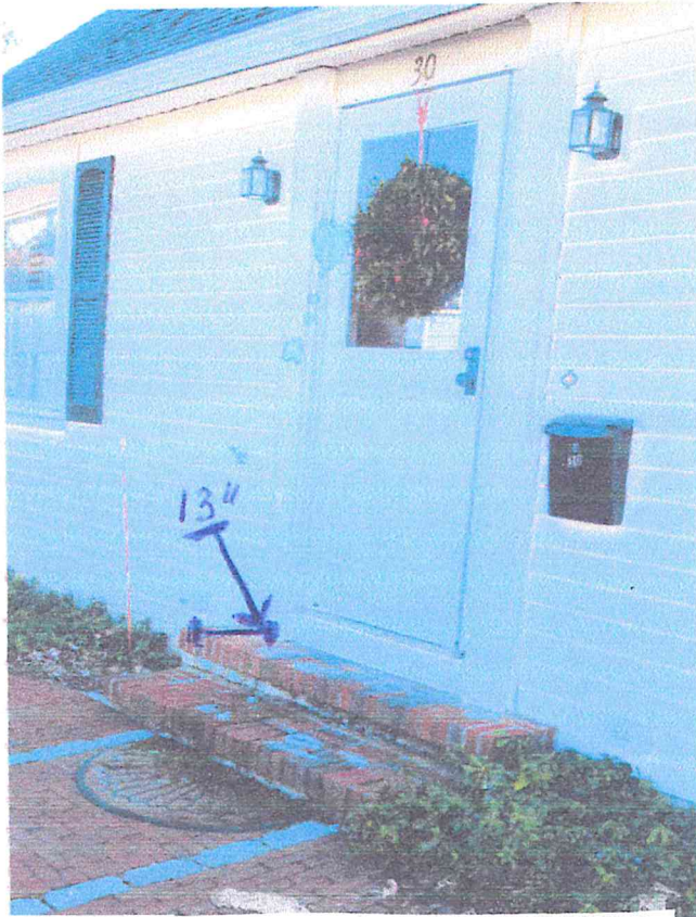
EXISTING entry at 30 Summer Street: Narrow (13" top, 15" bottom) brick steps. Total: 28" – No handrail.
