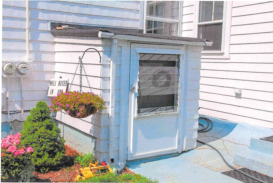
Photo 9 - Existing Doghouse Style Bulkhead Enclosure to be Removed and Replaced with Metal Bulkhead.
