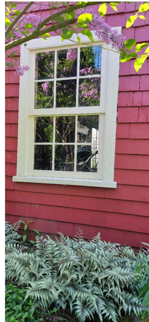
Photo #7: North double-hung 6-over-6 window
