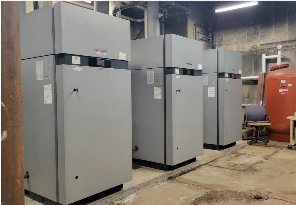
Three (3) natural gas furnaces located inside the boiler room.
