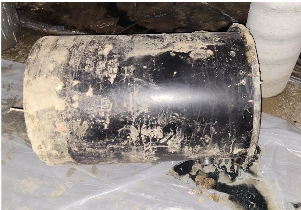
A chemical separator used to separate waste from the school's chemistry classes, which is located on the dirt floor of the basement.
