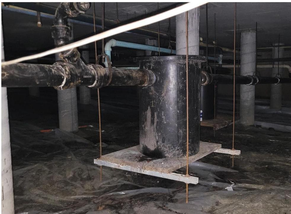
A chemical separator connected to the pipes which feed from the school's chemistry classes.
