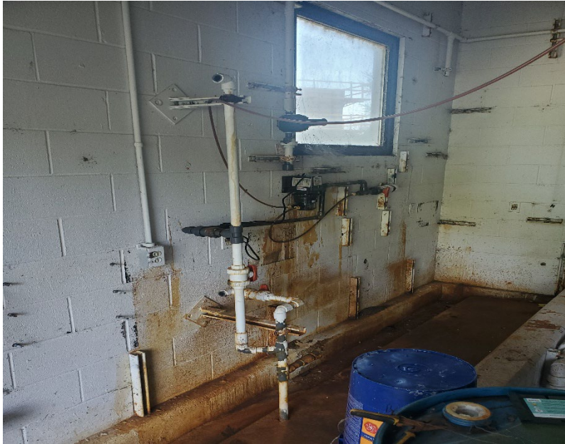
Pictures showing existing Ferric Chloride room and existing pump system
