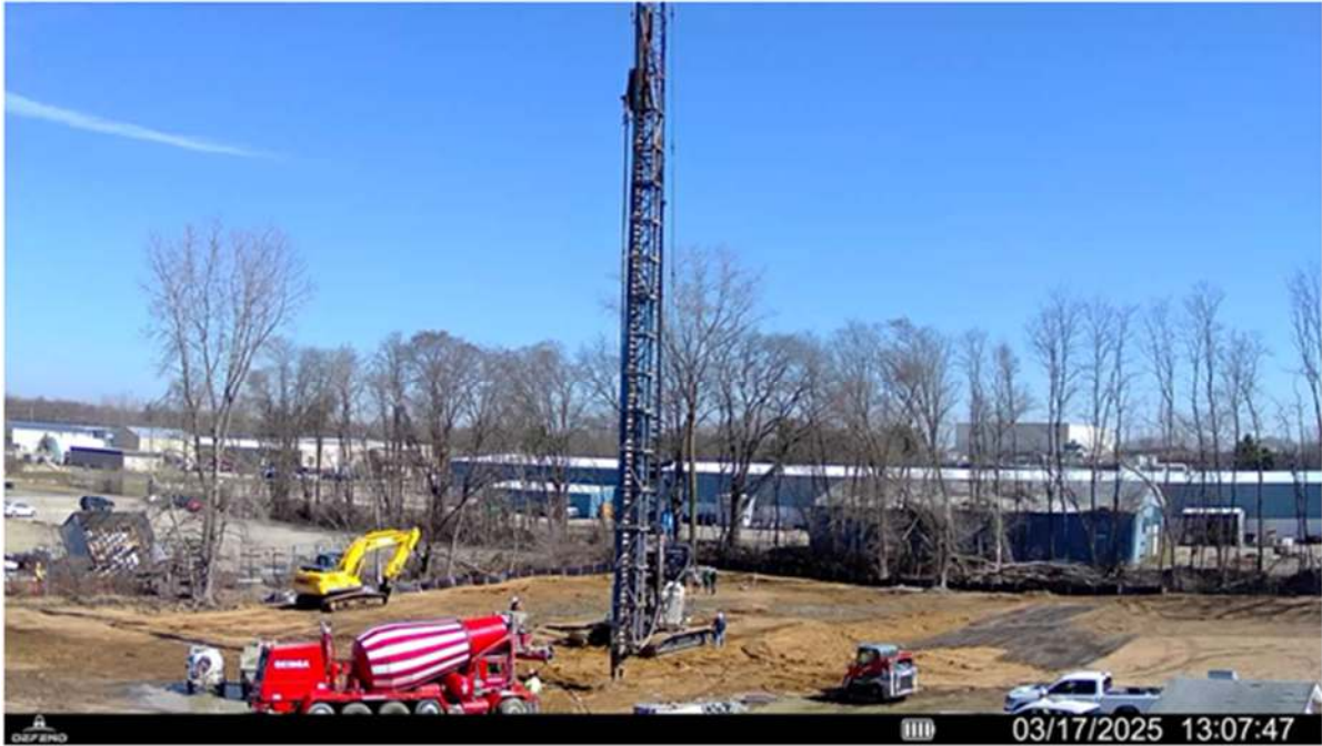
Water Tower drilling
