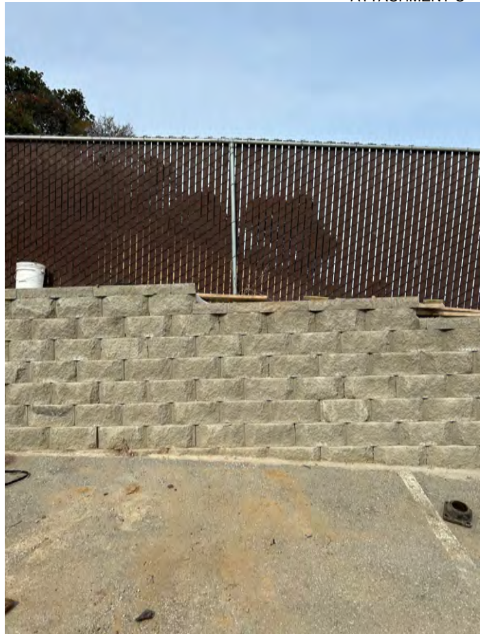
Existing brown-slatted fence and Allen-block retaining wall used throughout the site
