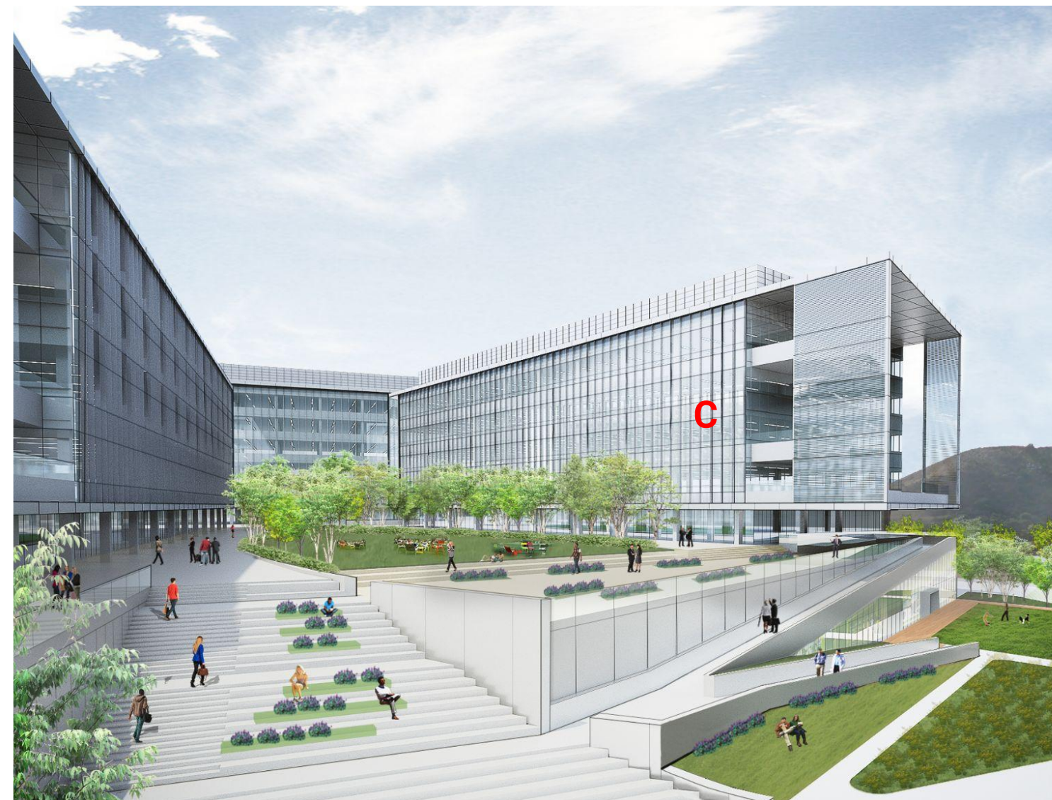
View from North looking at courtyard
