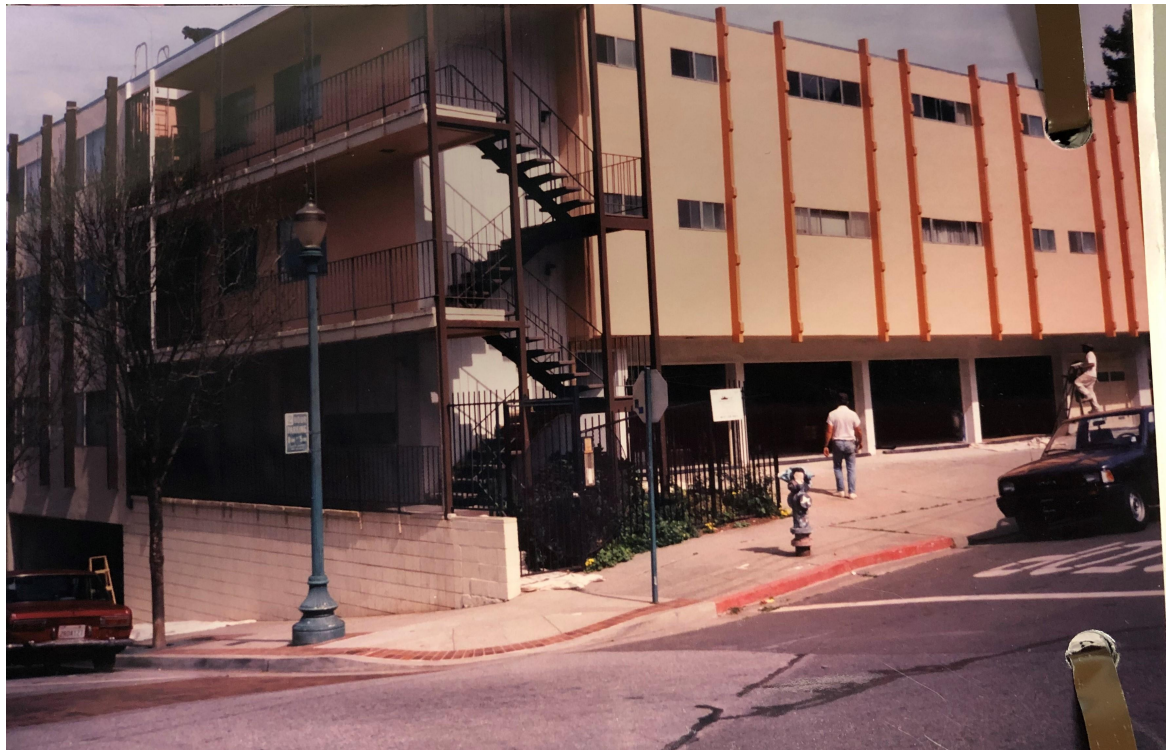
Building as originally constructed in the 1960s with an exterior staircase
