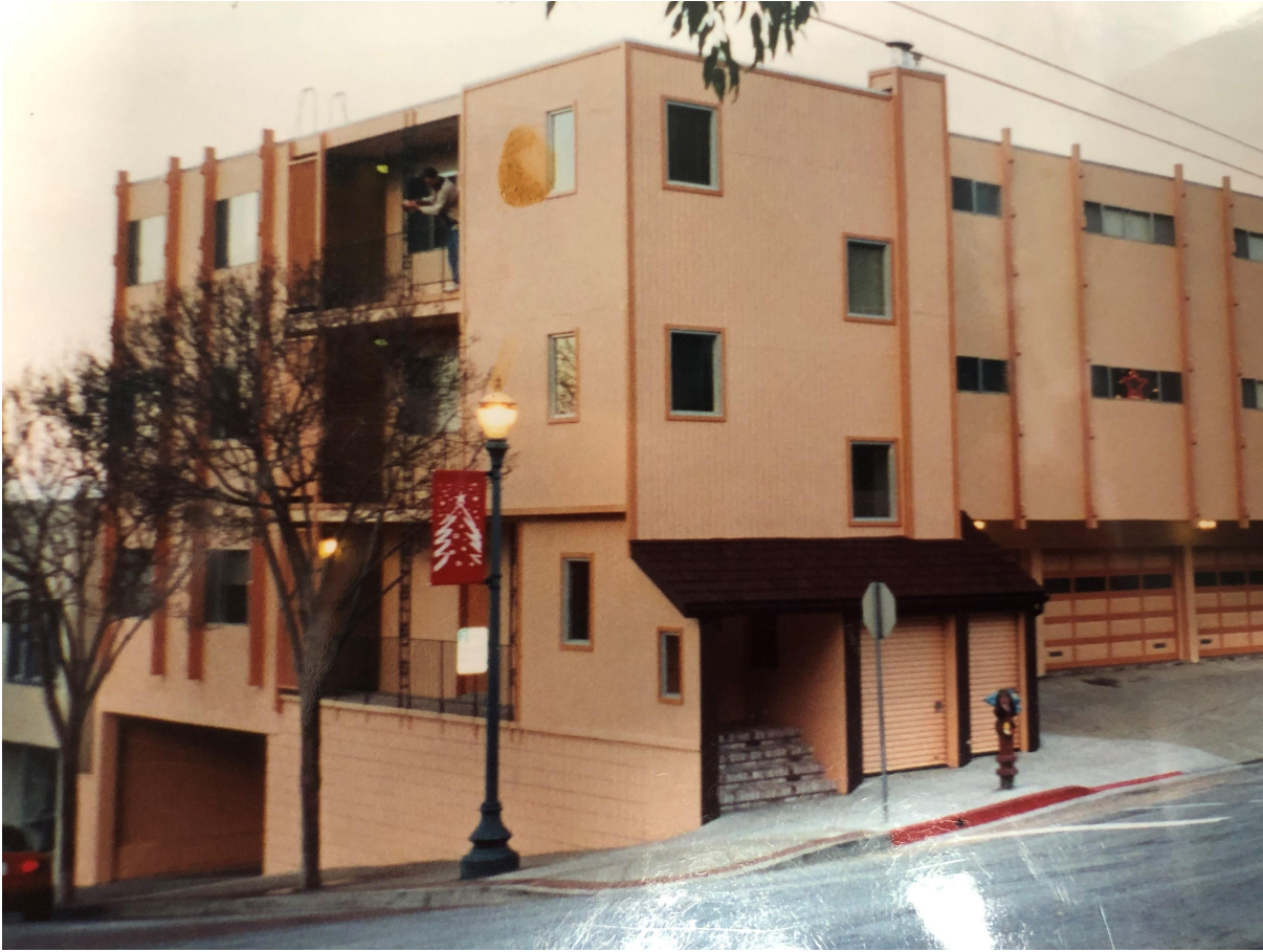
Building pre 2010 stucco refinish and post exterior stair enclosure
