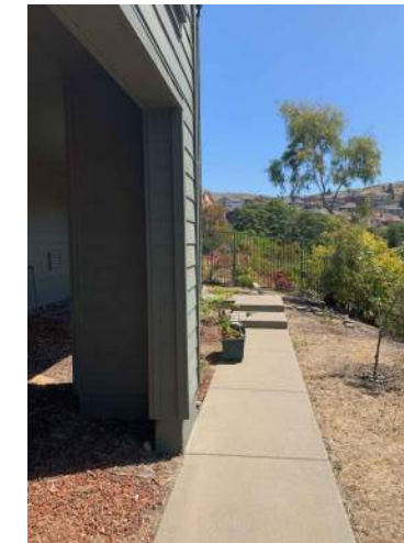
3 EXISTING CONCRETE PATHWAY I REMOVED & REPLACED
