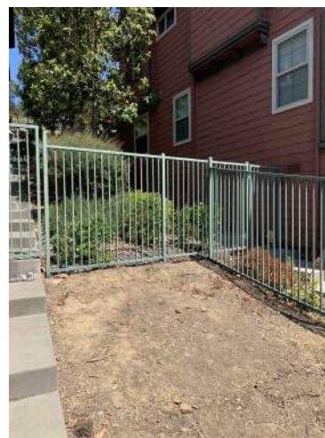
7 EXISTING FENCE & GATE AT SIDE YARD I TO REMAIN & PROTECT IN PLACE
