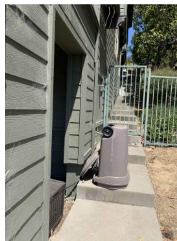
8 EXISTING CONCRETE STEP & ENTRY I REMOVED & REPLACED
