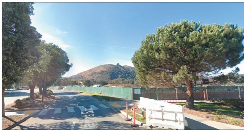
VIEW LOCATION 1 VIEW FROM NORTH WEST ALONG MARINA BLVD FACING FUTURE SITE OF 3000-3500 GENESIS MARINA
