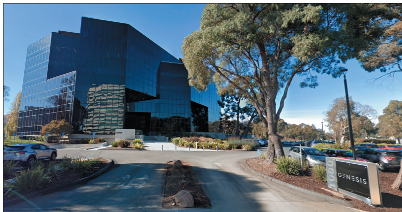
VIEW LOCATION 7 VIEW FROM MARINA BLVD PERPENDICULAR TO EXISTING SITE OF 1000 GENESIS VEHICULAR ENTRY
