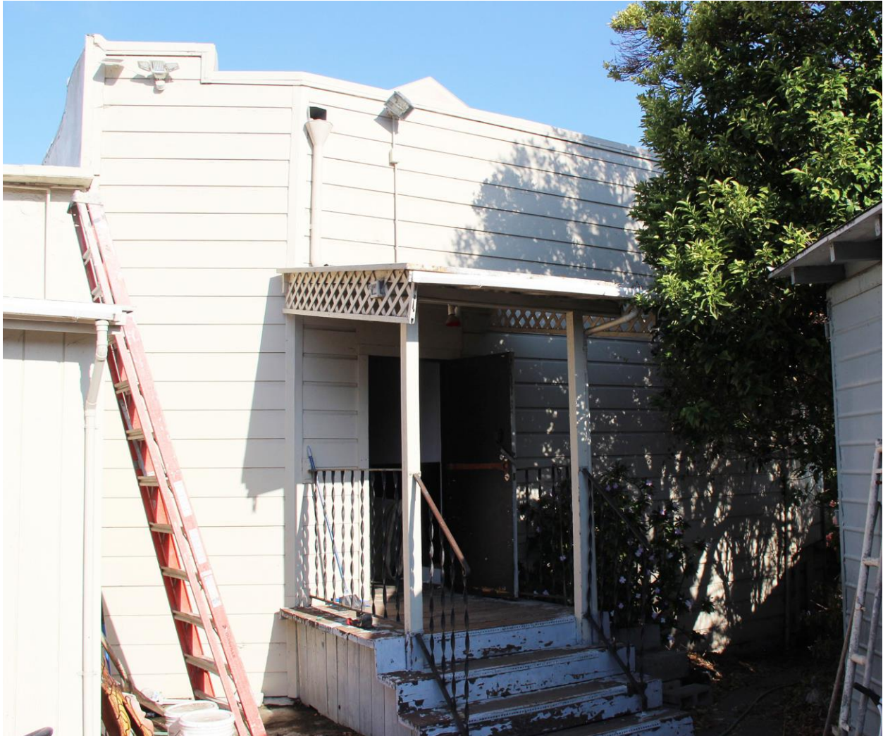
Figure 23. East (rear) façade of 23 Visitacion Avenue.
