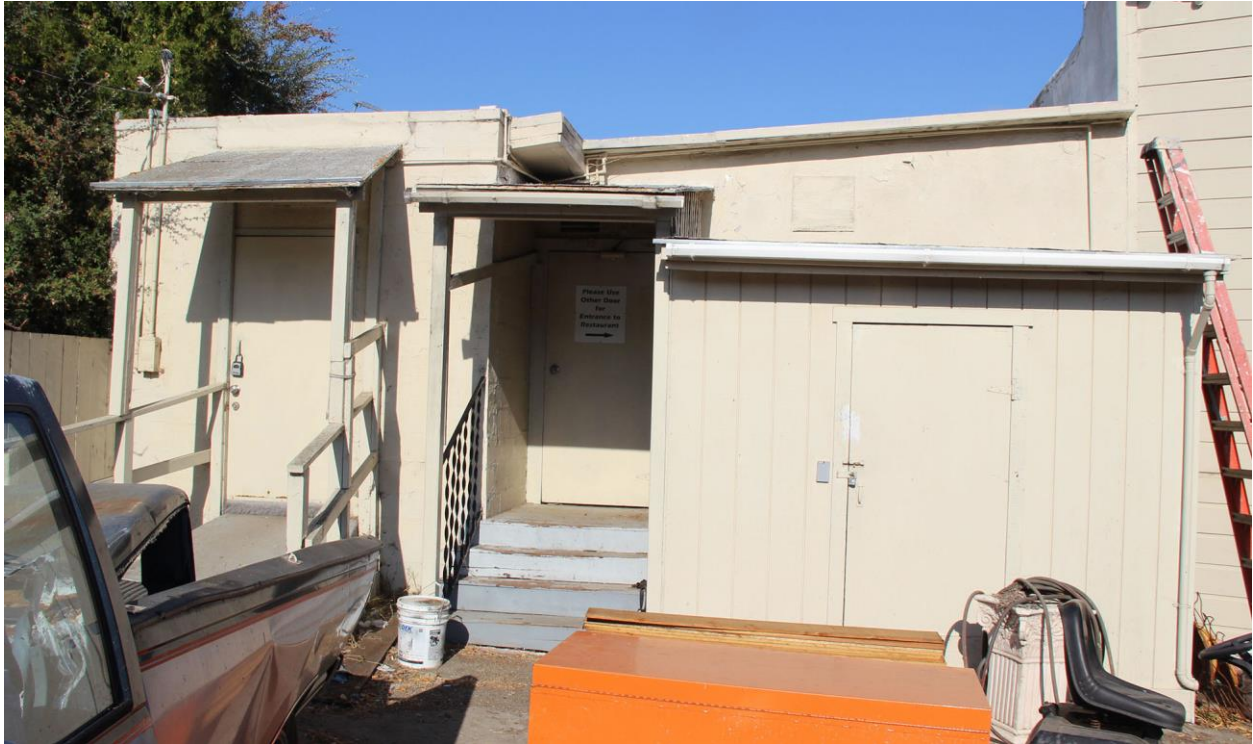
Figure 31. East (rear) façade of 25 Visitacion Avenue.
