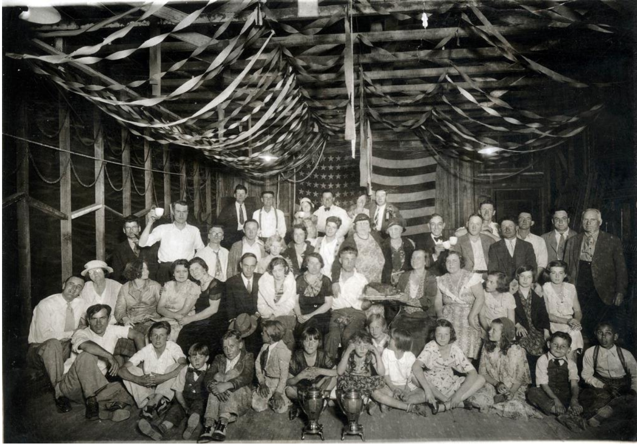
Figure 40. Interior of 23 Visitacion Avenue, Ca. 1935. Source: San Mateo County Library, Brisbane Library
