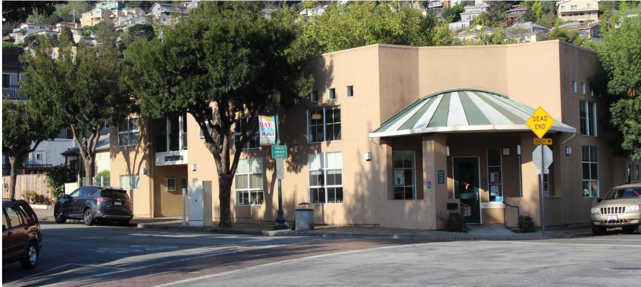
Figure 11. Visitacion Gardens, 2 Visitacion Avenue – built Ca. 2005.
