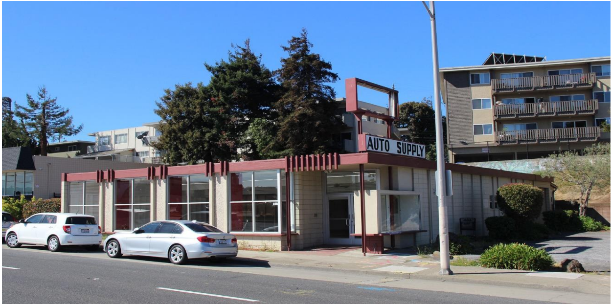
Figure 45. 321 El Camino Real, South San Francisco.
