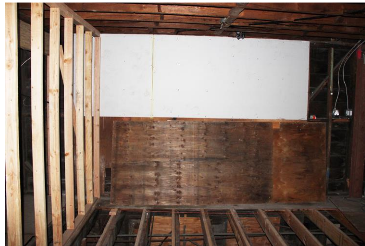
Figure 26. Bar area within interior of 23 Visitacion Avenue; view toward north.
