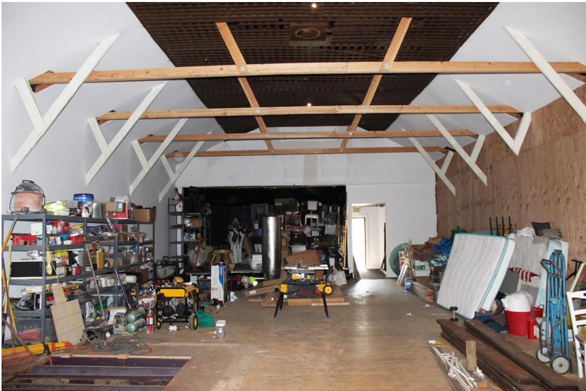
Figure 28. Auditorium of 23 Visitacion Avenue; view toward stage (east).
