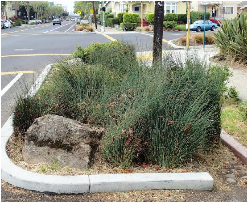
Bulbouts at key intersections should be built where feasible to reduce pedestrian crossing distances.
