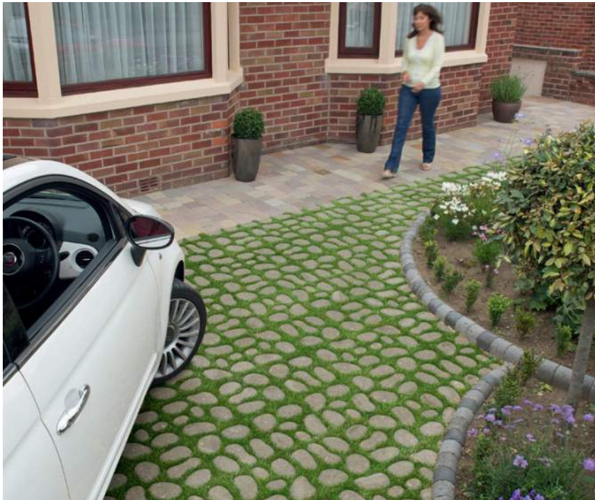
Permeable pavers should be incorporated to create an attractive and practical way to promote stormwater infiltration.
