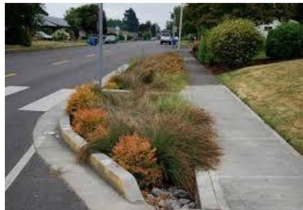
Sample Bioretention Basin Installed Along the Route
