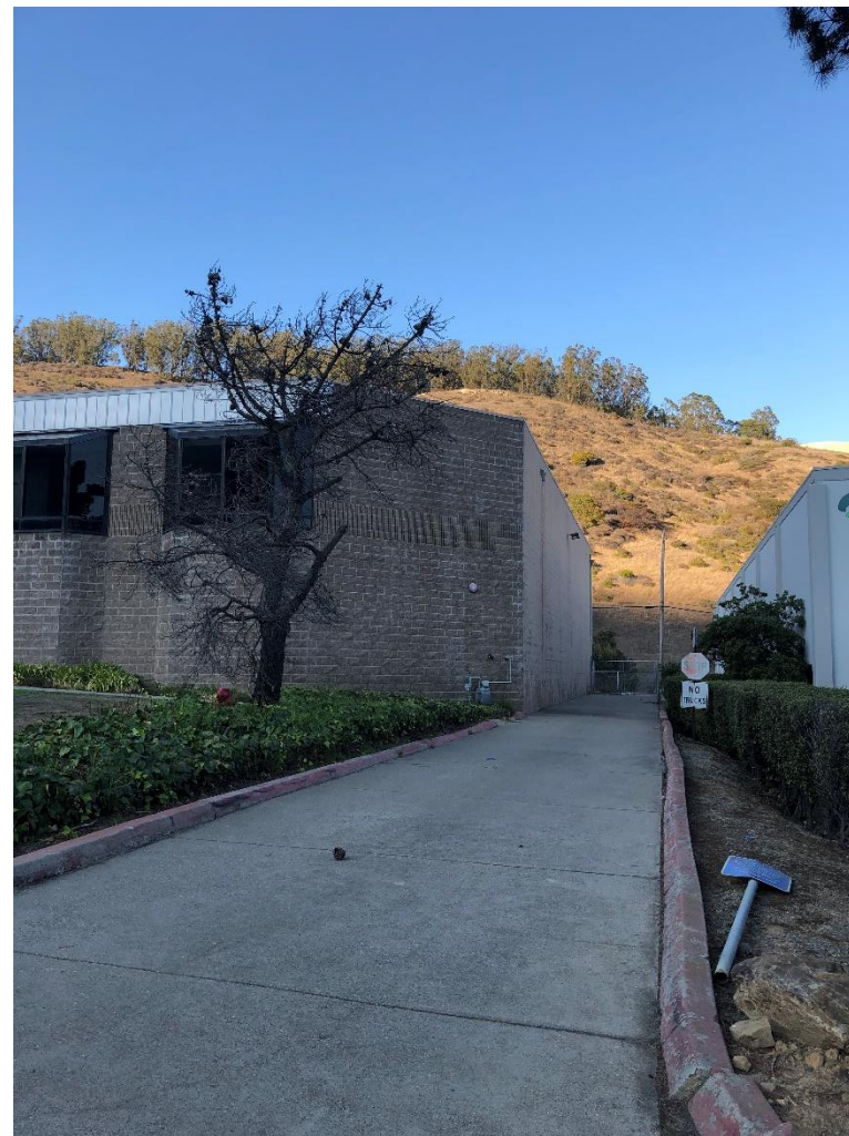
View of the eastern, entry driveway from W. Hill Pl.
