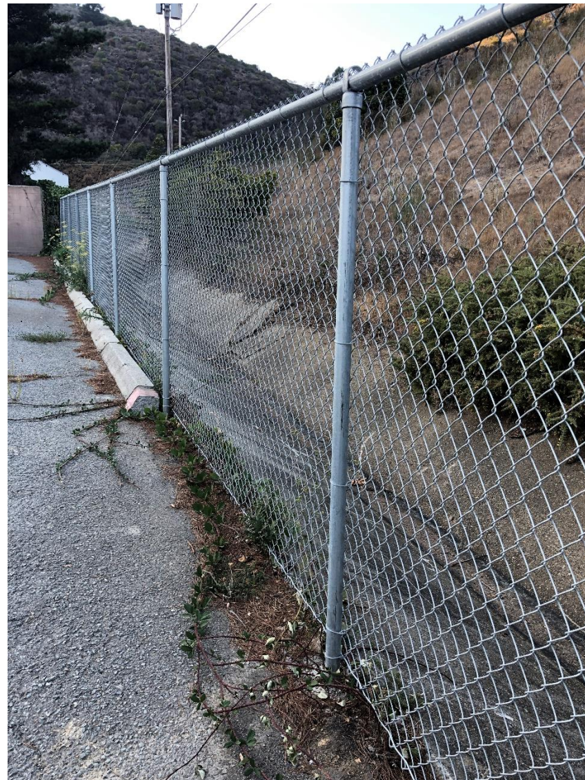
View of concrete v-ditch within City easement.
