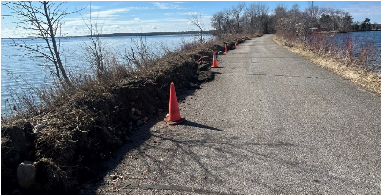
Figure 2: Shoreview Lane Existing Conditions - South Facing
