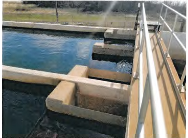
Olney Water Treatment Plant (2022)
