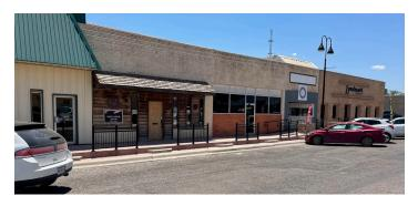
eHT provided project management and design for approximately 600 linear feet of new sidewalk on two blocks of the downtown square of Seminole. The project consisted of stamped concrete, colored concrete, handicap accessibility to all store fronts, planter boxes with irrigation, custom light poles, and custom railing and handicap ramps. The project utilized funds from the Texas Capital Fund.
