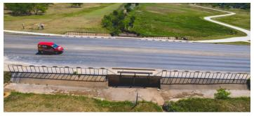
eHT is providing project management, design and construction administration for the replacement of aging roadway surface with full depth base, as well as drainage improvements along College Hills Boulevard (CHB). The project includes the rehabilitation of water and sewer utilities, roadway design, drainage evaluation and improvements, right-of-way verification, design survey, geotechnical investigation and the development of plans and specifications.
