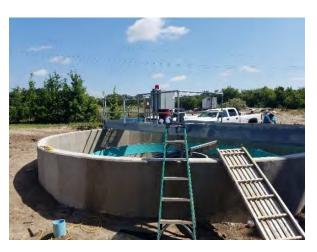
**Project Description:** Renovation of a 0.595 MGD wastewater treatment plant. The project included the construction of two new clarifiers, sludge drying beds, electrical, and appurtenances.
