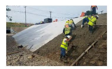
**Project Description**: Engineering design and construction administration for the Installation of approximately 540 square yards of concrete rip rap slope protection, paving, and incidentals.
