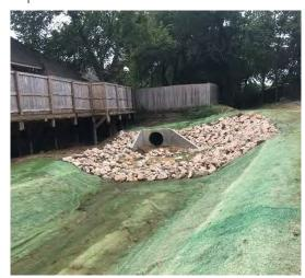
**Project Description**: Engineering design and construction administration for the Installation of approximately 2,700 square yards of grass lined drainage channel, and incidentals.
