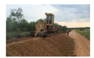
**Project Description**: Engineering design and construction administration for the Installation of an intake structure on Mill Creek and approximately 70,000 LF of 10" raw water supply line. **JM** also assisted with an amendment to the San Saba water rights for withdraw of water from Mill Creek at an alternative take point.
