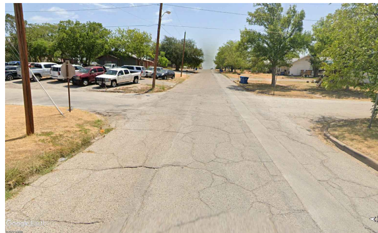
SMITH ST INTERSECTION
