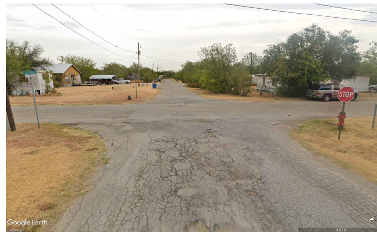
HARVEY ST INTERSECTION
