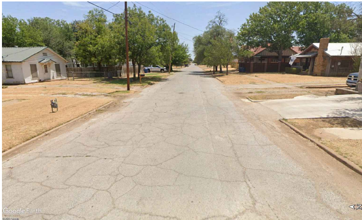
BETWEEN OAKWOOD ST AND SHELTON ST
