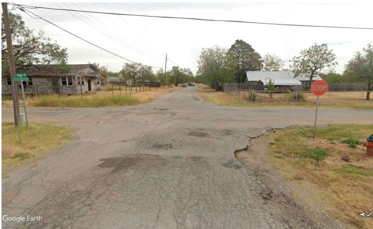
HARVEY ST INTERSECTION
