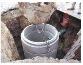
**Project Description**: Engineering design and construction administration for the Installation of approximately 2,500 linear feet of 8" and 6" PVC sewer lines including all manholes, bore and encasement, pavement repair, and incidentals.
