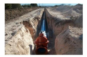
**Project Description**: Engineering design and construction administration for the Installation of a new raw water pump station and head tank located at Hords Creek Lake, approximately 44,000 LF of 16" raw water supply line and approximately 40,000 linear feet of water distribution lines.
