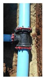
**Project Description**: Engineering design and construction administration for the Installation of approximately 20,360 linear feet of 12" Thru 1" water line, valves, fittings, water line connections, service re-connections, bore & encasement, and incidentals
