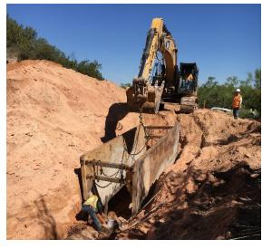
**Project Description**: Engineering design and construction administration for the replacement of approximately 1,500 linear feet of 30 "sewer line and manholes.
