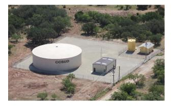
**Project Description**: Engineering design and construction administration for the Installation of a 2 MGD pump station and 1.0 MG wire-wound, pre-stressed concrete ground storage tank.
