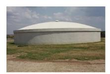
Project Description: Engineering construction design and administration for the Installation of 8 MGD pump station and 2.0 MG wire-wound, pre-stressed concrete ground storage tank.
