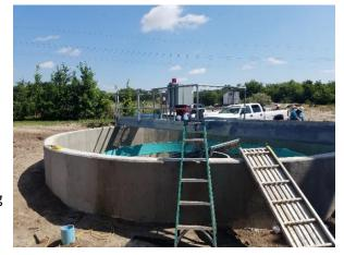
**Project Description:** Renovation of a 0.595 MGD wastewater treatment plant. The project included the construction of two new clarifiers, sludge drying beds, electrical, and appurtenances.
