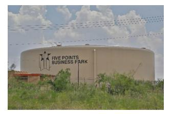
**Project Description**: Engineering design and construction administration for the re-construction of the roof and recoating of the interior and exterior of a 7.5 MG welded steel ground storage tank.
