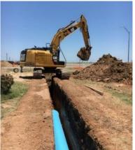
**Project Description**: Engineering design and construction administration for the Installation of approximately 19,000 linear feet of 6'' - 18'' PVC water lines including all valves, fittings, water line connections, bore and encasement, pavement repair
