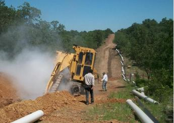
**Project Description**: Engineering design and construction administration for the Installation of approximately 40,000 LF of 24" treated water supply line.
