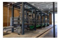
**Project Description:** 4.5 MGD Surface Water Treatment Plant Improvements The project included an evaluation of existing treatment efficiencies and alternatives for new treatment techniques. This project also included a pilot study of multiple membrane filtration vendors and construction of a 4.5 MGD membrane ultrafiltration system and new Water Treatment Plant. The project also included the construction of a new high service pump station as well as a new chemical storage facility.
