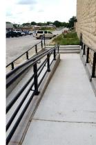
**Project Description**: Engineering design and construction administration of 600 SY of concrete sidewalk reconstruction, including ramps, curb ang gutter, and street lighting
