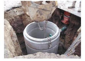
**Project Description**: Engineering design and construction administration for the installation of approximately 5,000 linear feet of 8" PVC sewer lines including all manholes, bore and encasement, pavement repair, and incidentals and lift station improvements.
