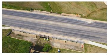
eHT provided project management, design, and construction administration for the replacement of aging roadway surface with full depth base, as well as drainage improvements along College Hills Boulevard (CHB). The project included the rehabilitation of water and sewer utilities, roadway design, drainage evaluation and improvements, right-of-way verification, design survey, geotechnical investigation, and the development of plans and specifications.
