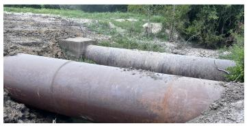
eHT provided project management, design, and construction administration for an upgrade of approximately 4.6 miles of trunk main that serves the AJ Brown Wastewater Treatment Plant (WWTP), owned and operated by the City of Huntsville. The project included the installation of approximately 1.1 miles of 48-inch PVC sewer line and 3.5 miles of 42-inch PVC sewer line. The project also included approximately 72 pre-cast concrete manholes and 15 branch connections.
