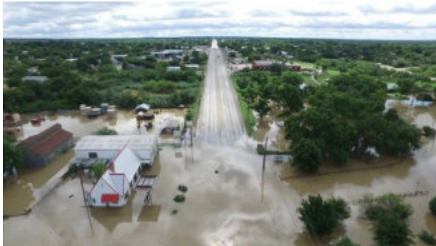
Photo 1: Flooding on US180 East near City Park (KTXS News Photo)
