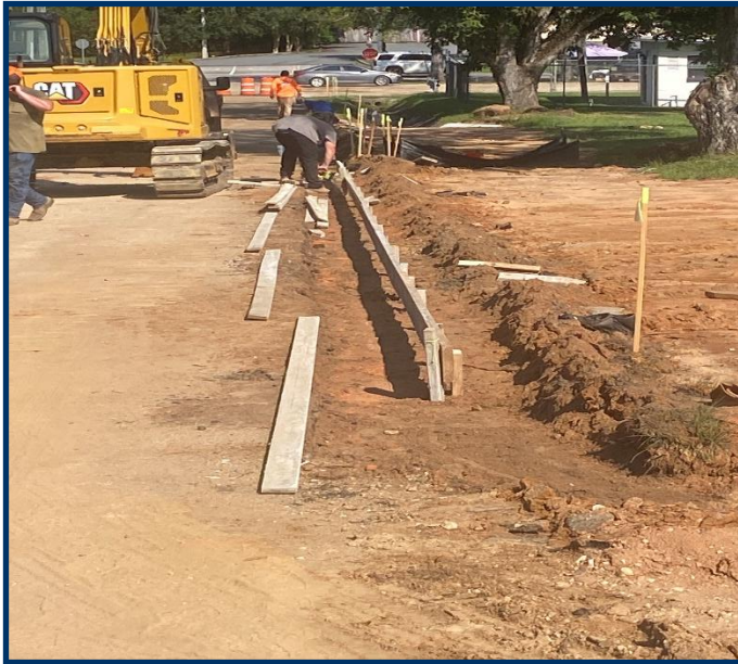
Bonifay Memorial Field Drainage Improvements Subcontractor building form for curb and gutter on Veterans Blvd. RT side per plans.
