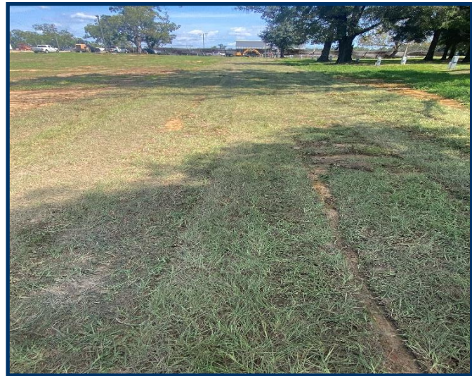
Bonifay Memorial Field Drainage Improvements Contractor installed Performance Turf Sod in field between Depot St. and McGee St.
