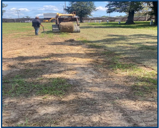
Bonifay Memorial Field Drainage Improvements Contractor installed Performance Turf Sod between Depot St. and McGee St.
