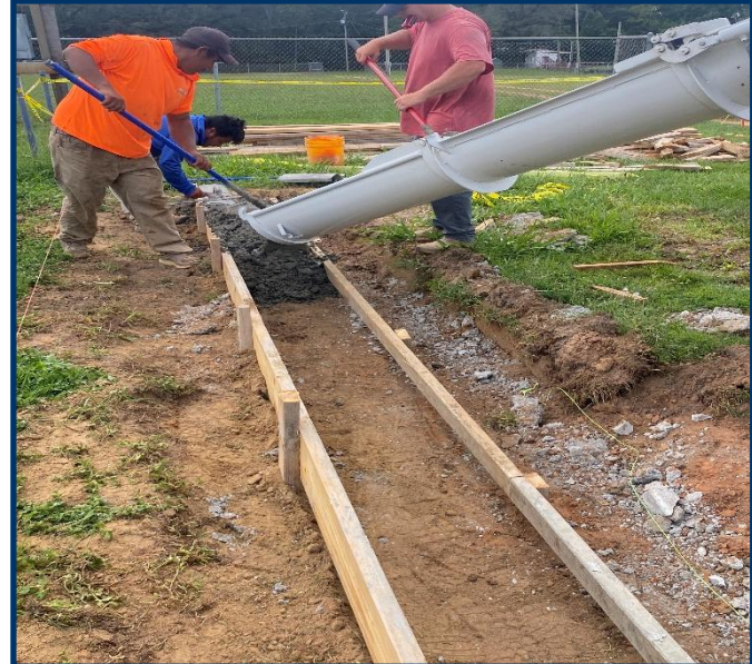
Bonifay Memorial Field Drainage Improvements Subcontractor installing NS concrete for curb and gutter in Southside Parking Area per plans.
