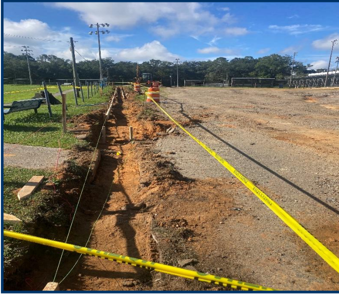
Bonifay Memorial Field Drainage Improvements Subcontractor building form for curb and gutter in Southside Parking Area per plans.
