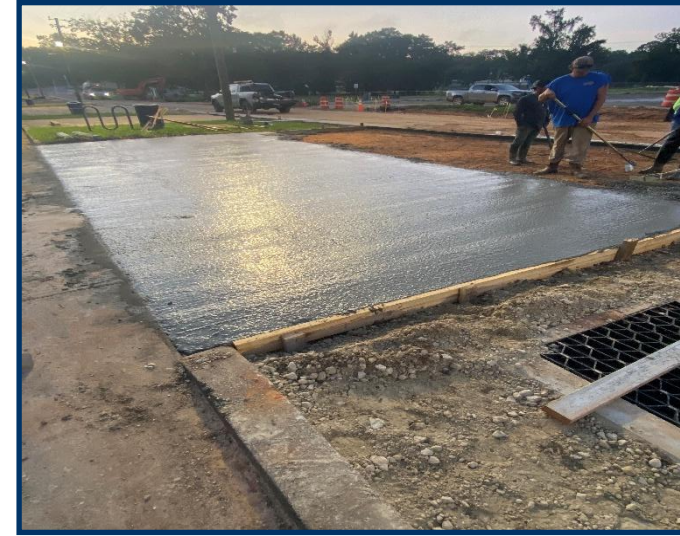
Bonifay Memorial Field Drainage Improvements Contractor installed and compacted select fill at Sta. 26+94 to 27+94 RT side.
