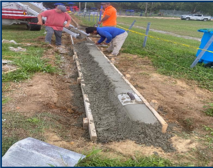
Bonifay Memorial Field Drainage Improvements Subcontractor installing NS concrete for curb and Gutter in Southside Parking Area per plans.
