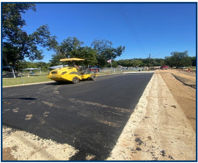
Bonifay Memorial Field Drainage Improvements Contractor installed and compacted SP 12.5 Asphalt in parking bay on Northside of Veterans Blvd.
