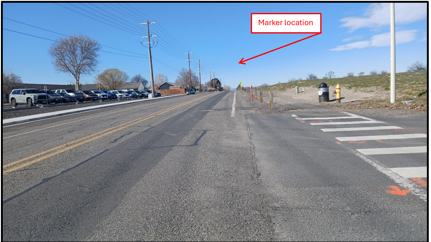
Figure D: Anthony Access – Looking from 500 feet East
