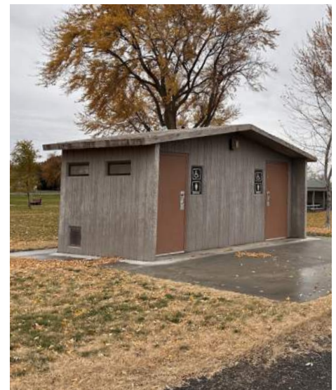
Upgrade Existing Restrooms
