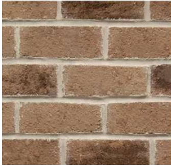
Walls / Columns Old Georgetown Material: Brick
