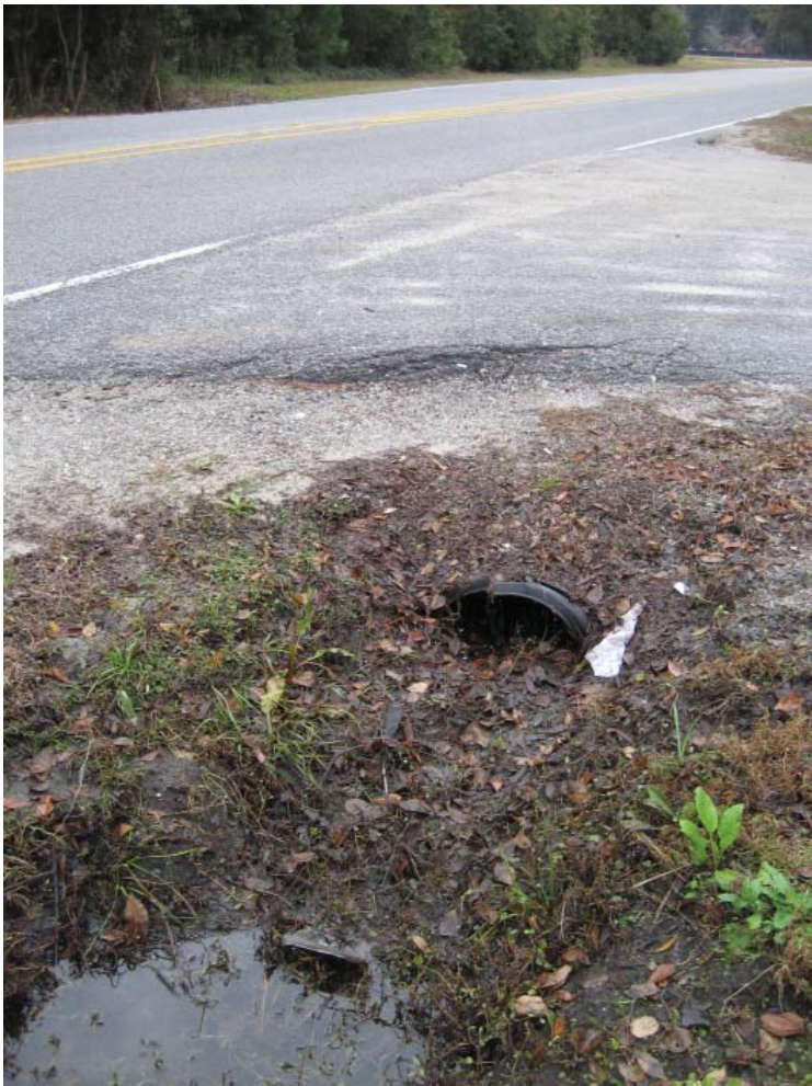
Figure 80: Typical clogged culvert found along the roadways.
