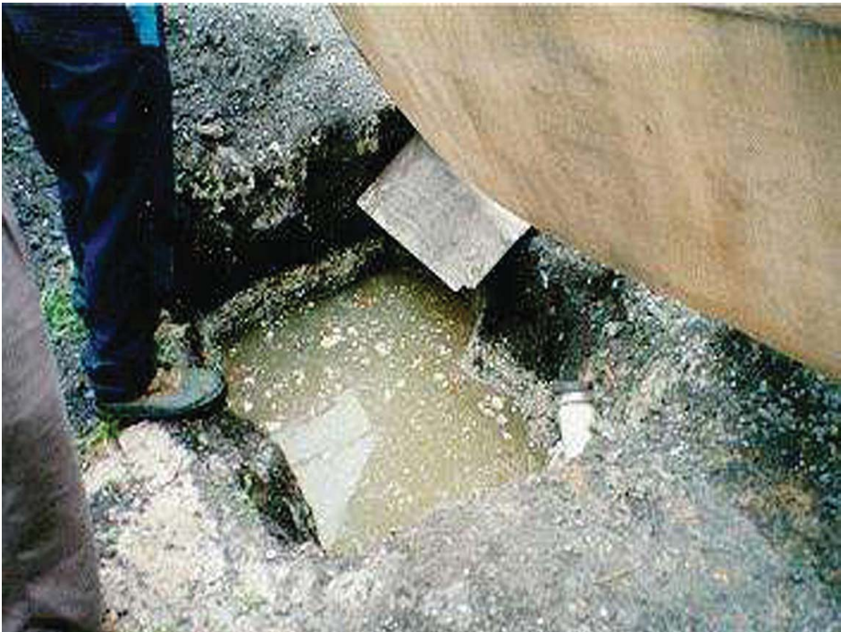
Figure 35: Failing septic tank.
