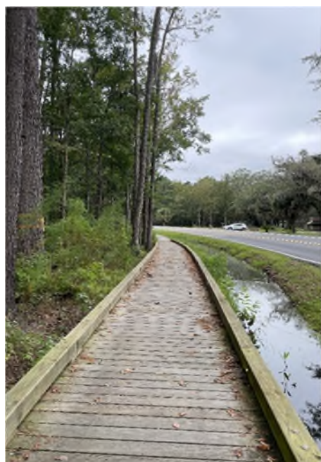
At the request of the residents, handrails were installed on this Buck Island Road boardwalk for additional safety. See cover photo for post-installation view.
