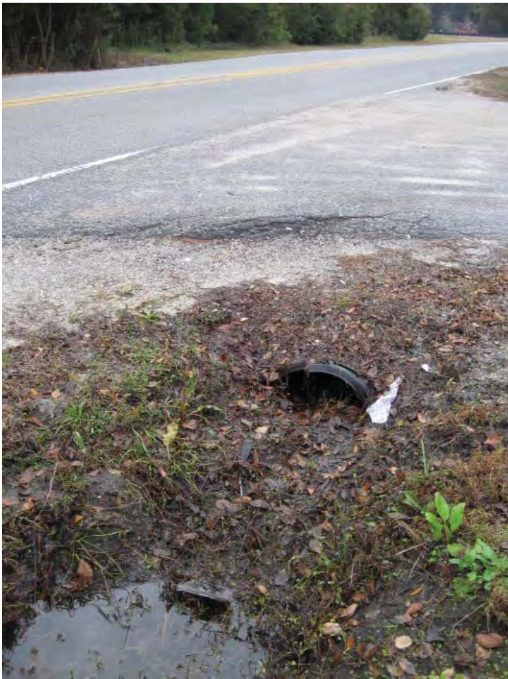
Figure 80: Typical clogged culvert found along the roadways.
