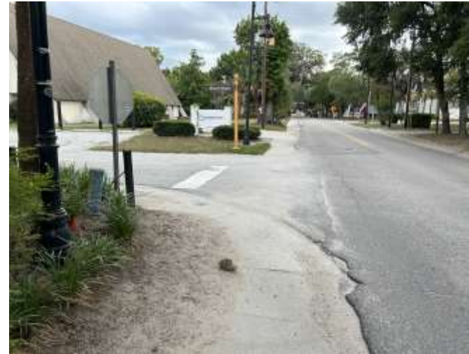
No Curb / Poor Drainage – Limited Driveway Aprons
