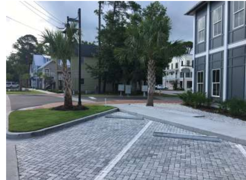
Angled Paver Parking with Raised Curb and Sidewalk
