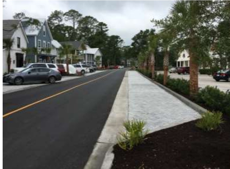
Parallel Paver Parking with Raised Curbs and Valley Gutter
