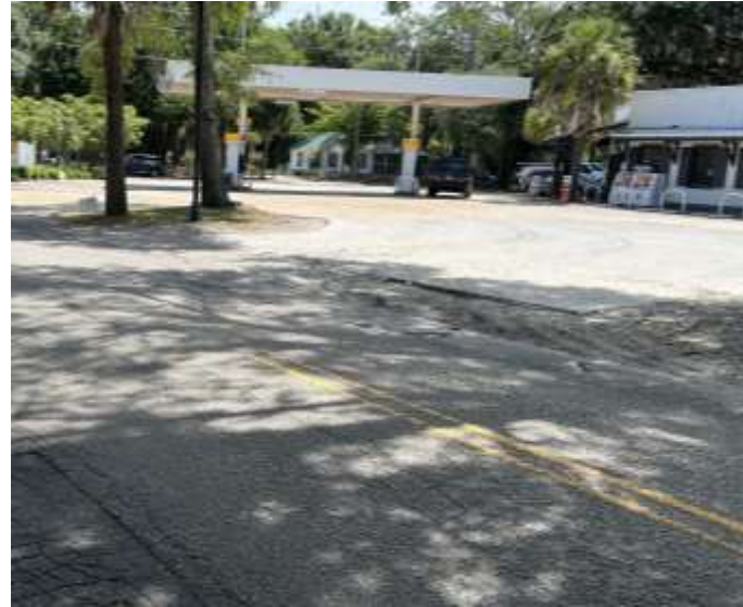
Poor Pavement Condition – Potholes and Rutting
