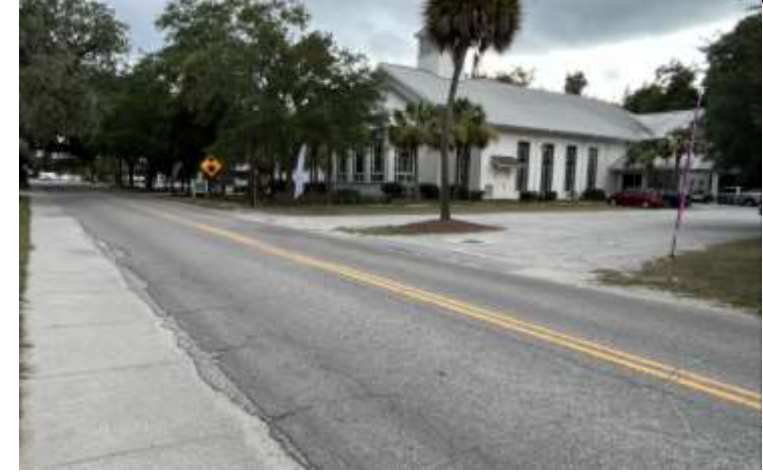
No Curb / Poor Drainage – Limited Driveway Aprons
