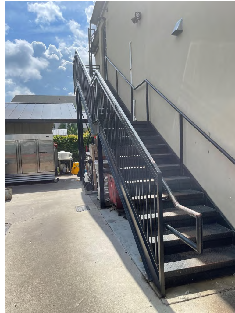
STAIR AT REAR OF BUILDING
