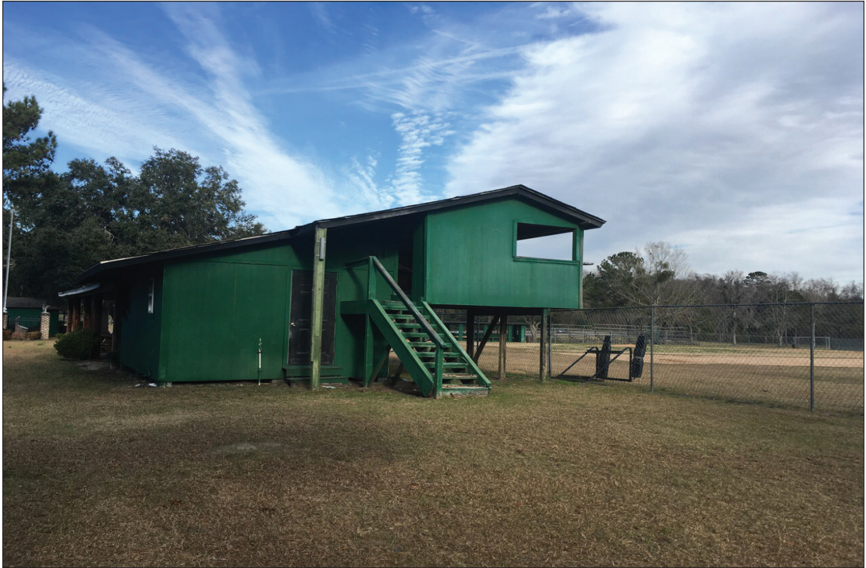
Figure 5.3 Eagles Field, facing northeast.
