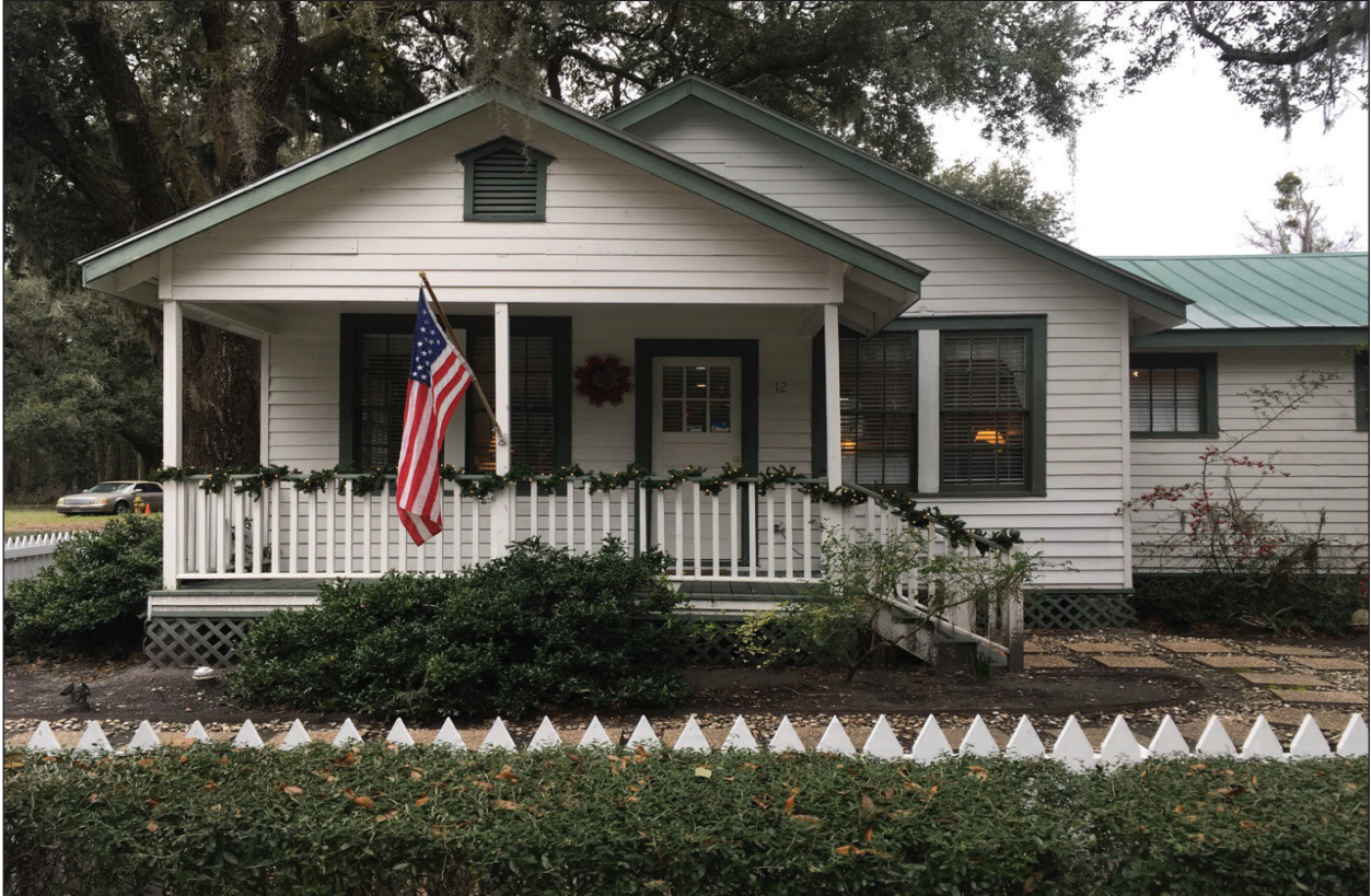
Figure 4.10 Example of a gable-front house within the Bluffton Historic District Survey Area featuring a projecting front porch (Resource 046-109, the Simmons-Joiner House, 12 Bruin Rd.).
