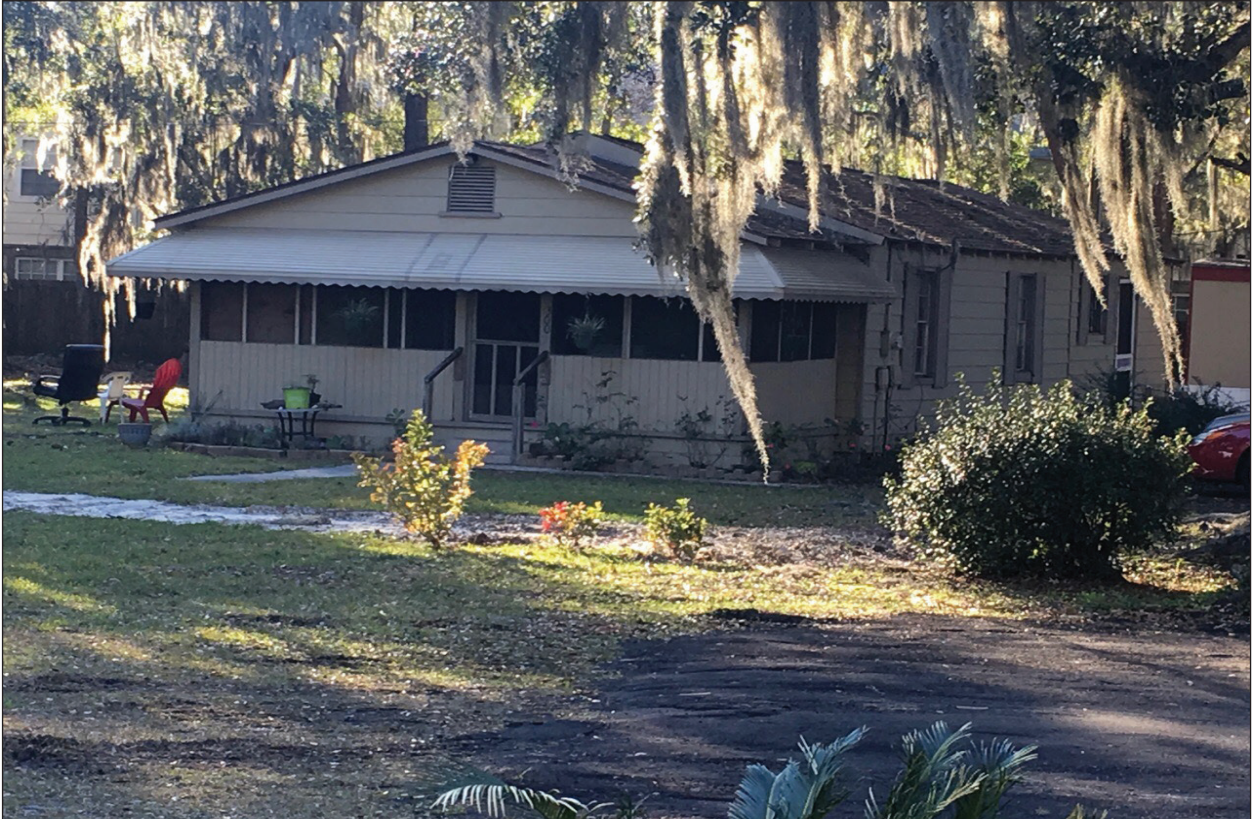
Figure 4.12 Example of a gable-front house within the Buck Island-Simmons ville Survey Area featuring exposed rafter tails, suggesting a Craftsman influence (Resource at 5238, 300 Buck Island Rd.).
