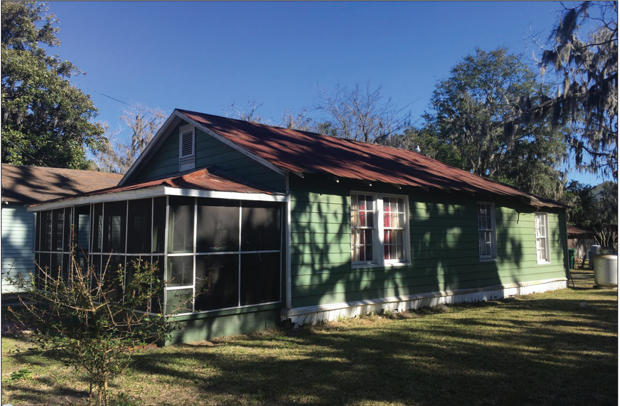
Figure 4.11 Example of a gable-front house within the Bluffton Historic District Survey Area featuring exposed rafter tails, suggesting a Craftsman influence (Resource 046-0062, 5 Calhoun St.).
