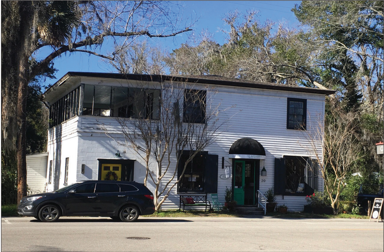
Figure 4.23 Constructed c. 1890 and long served as a general store. Residents recall both black and white Blufftonians shopping in the store. There is a private residence above the shop. This resource is within the Bluffton Historic District Survey Area (Resource 046-0065, Planter's Mercantile, 20 Calhoun Street).
