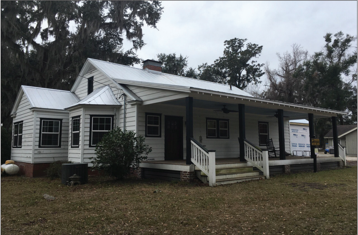
Figure 4.13 Example of a side-gabled house constructed in 1939 within the Bluffton Historic District Survey Area (Resource 046-0056, 40 Colcock Street).
