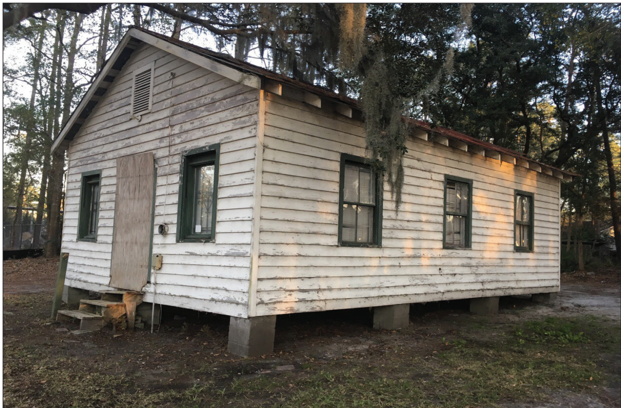
Figure 5.1 First Zion Baptist Church (Resource 5016), facing northeast.
