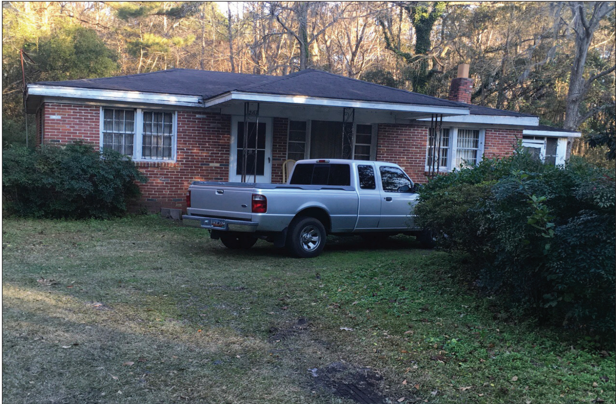
Figure 4.22 Example of a hip-roofed Ranch house with original wooden windows within the Buck Island-Simmons ville Survey Area (Resource 5235, 261 Buck Island Road).
