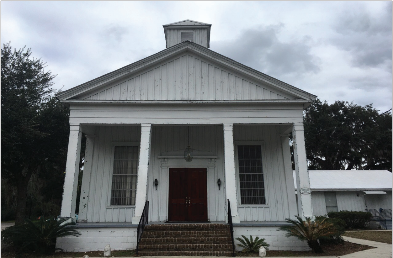
Figure 4.34 Resource 046-0087, Campbell Chapel AME Church, 23 Boundary Street, is one of two individually listed resources in the survey area. This church has elements of the Greek Revival style, including the pedimented front gable.
