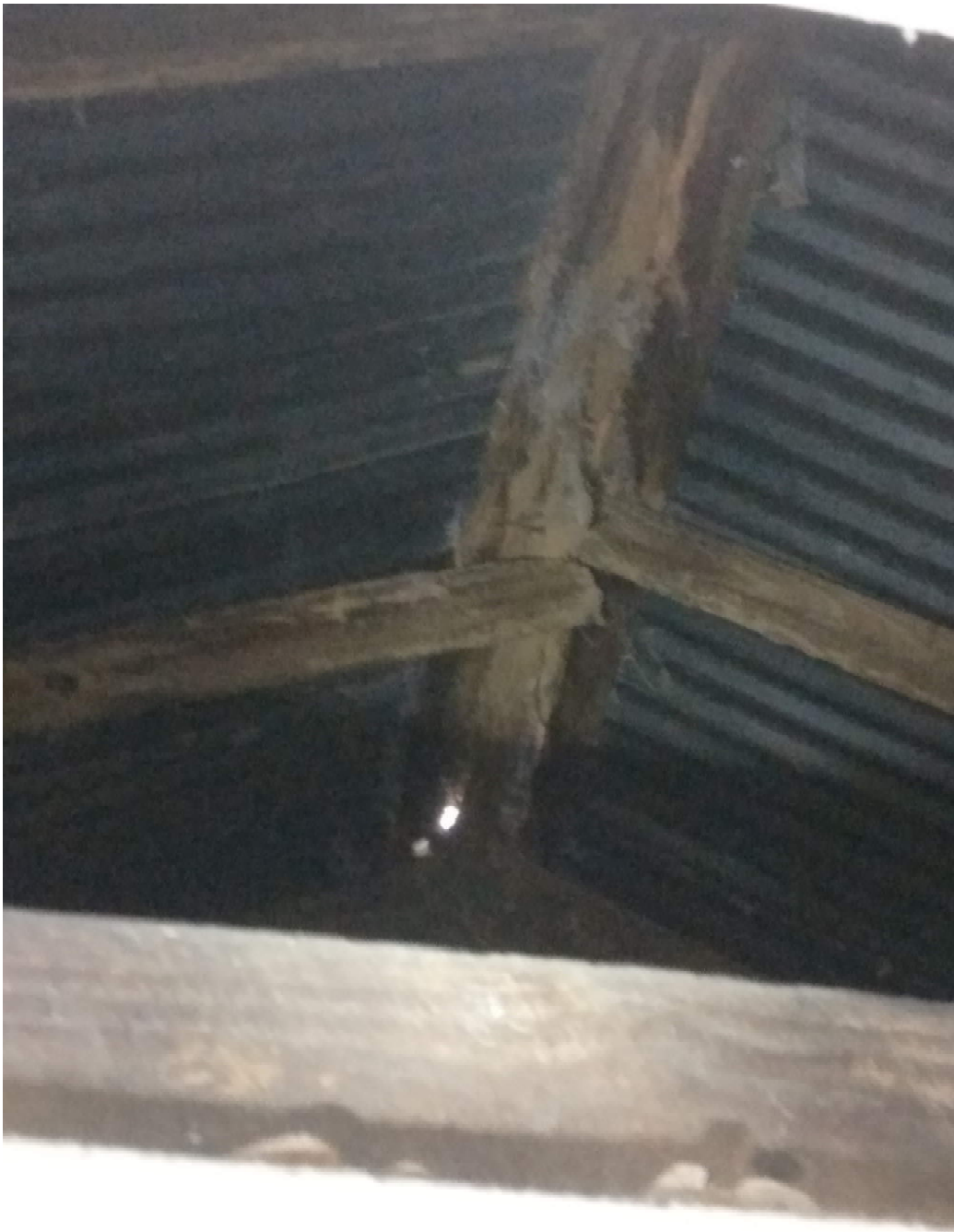
Roof Rafters not connected to ridge board
