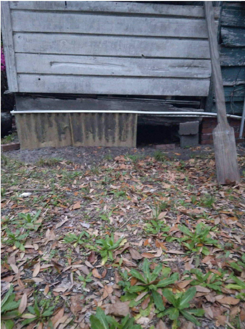
South West Porch Supports Broken CMU Block due to incorrect orientation
