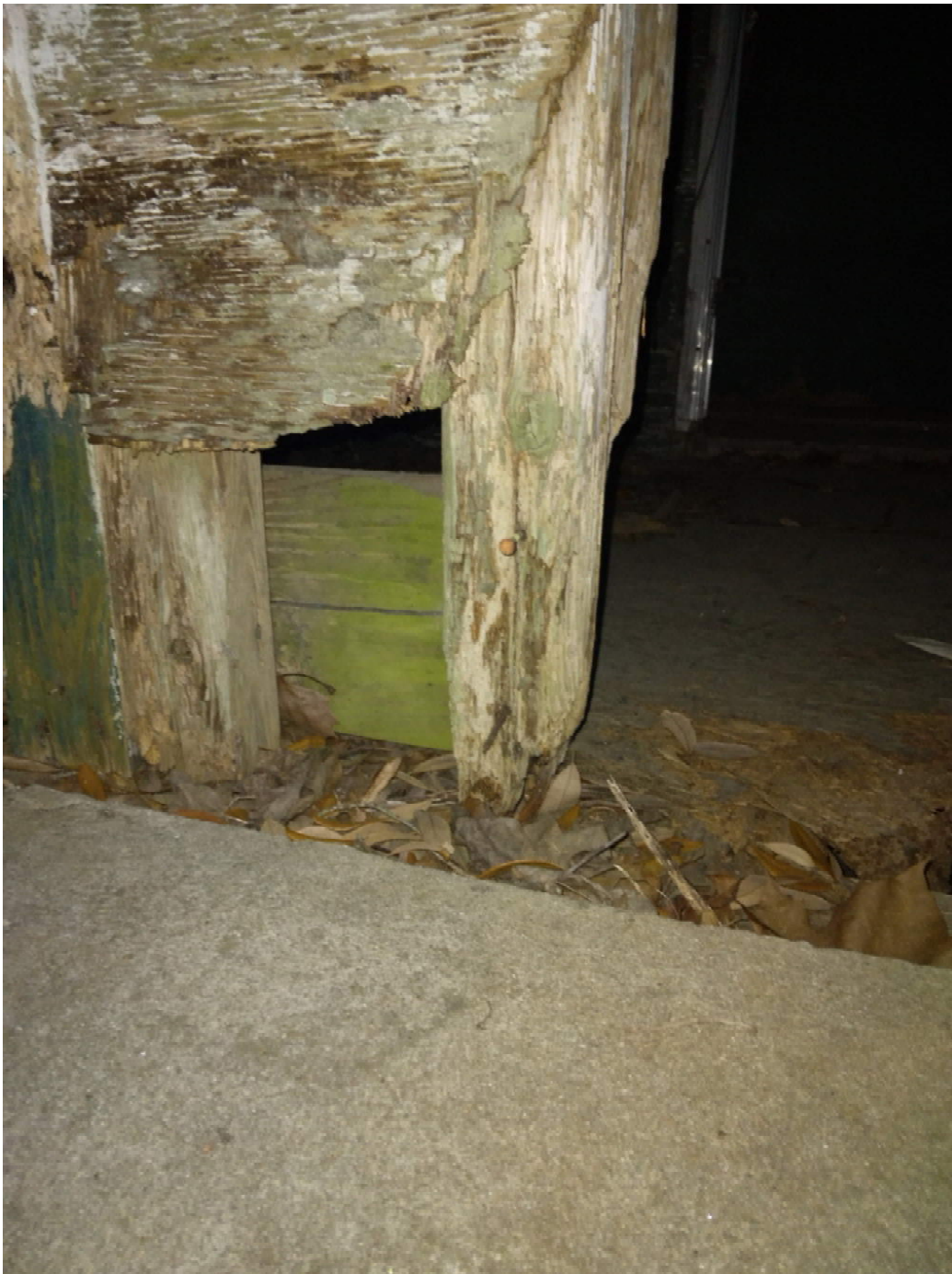
Rotten Jack and King post at Porch door
