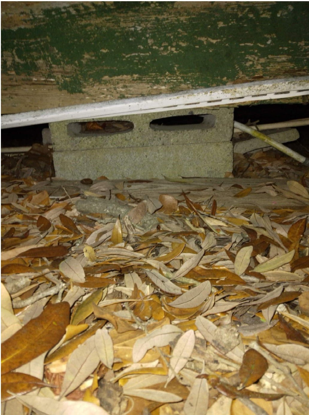
Incorrect loading of 4" CMU block
