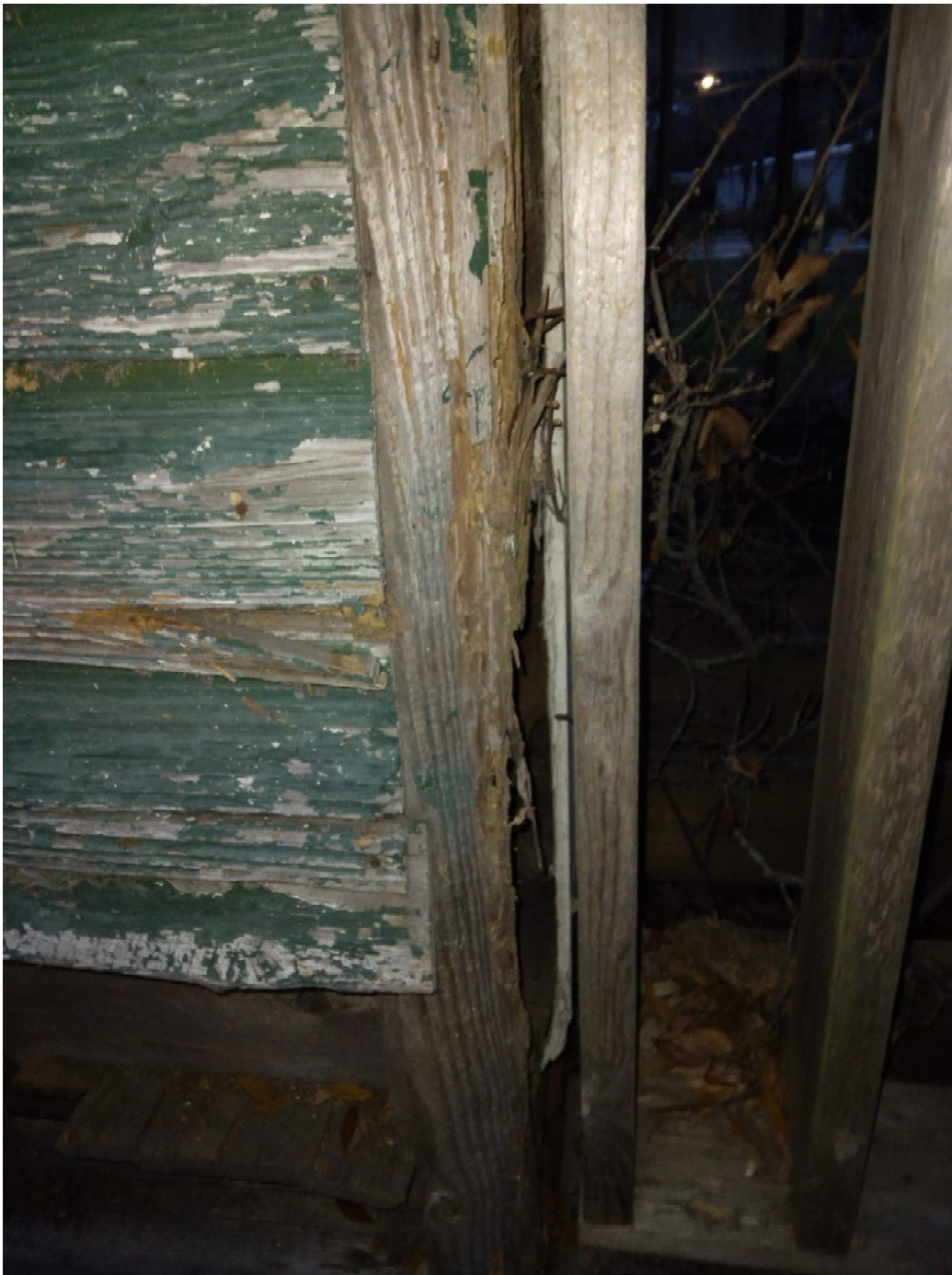
North West Corner finish rotten
