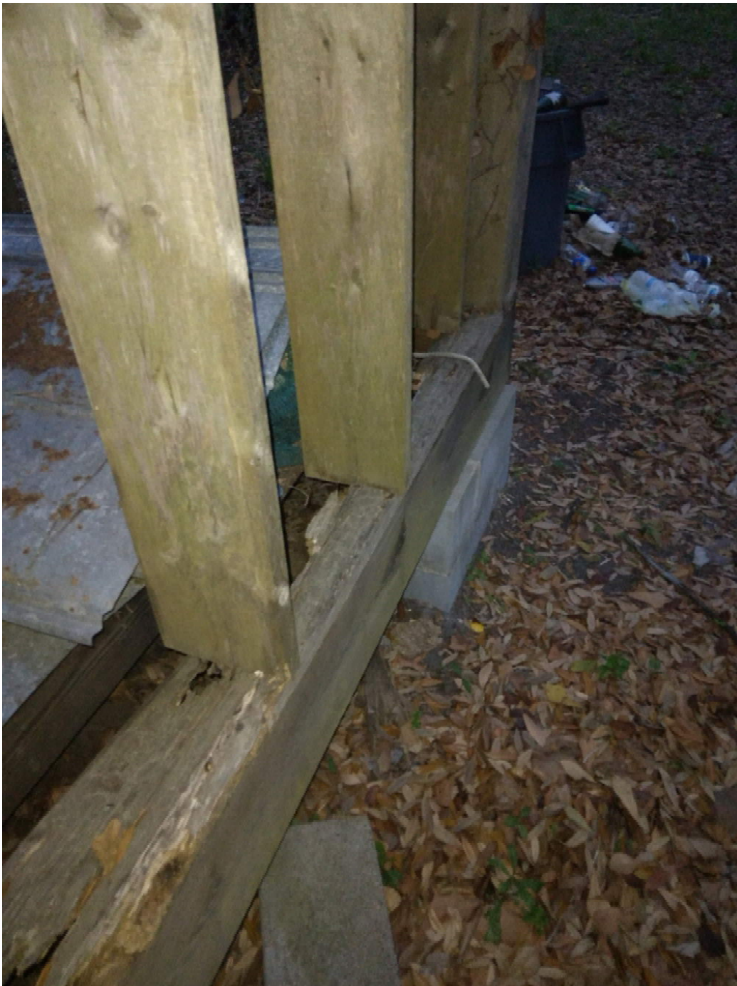
Back Room with rotten shoe plate and studs
