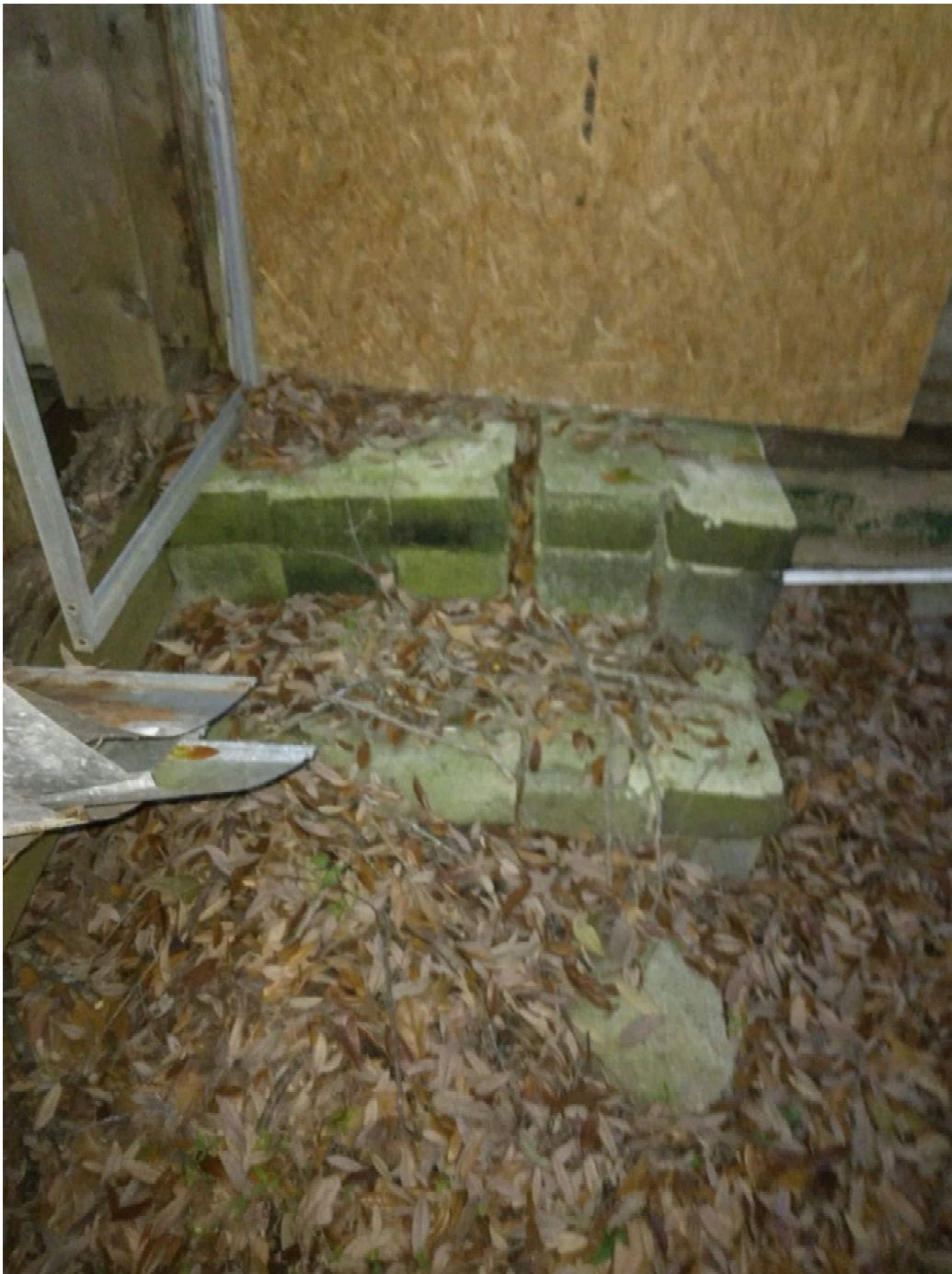
Back Entrance Stair construction is not to code
