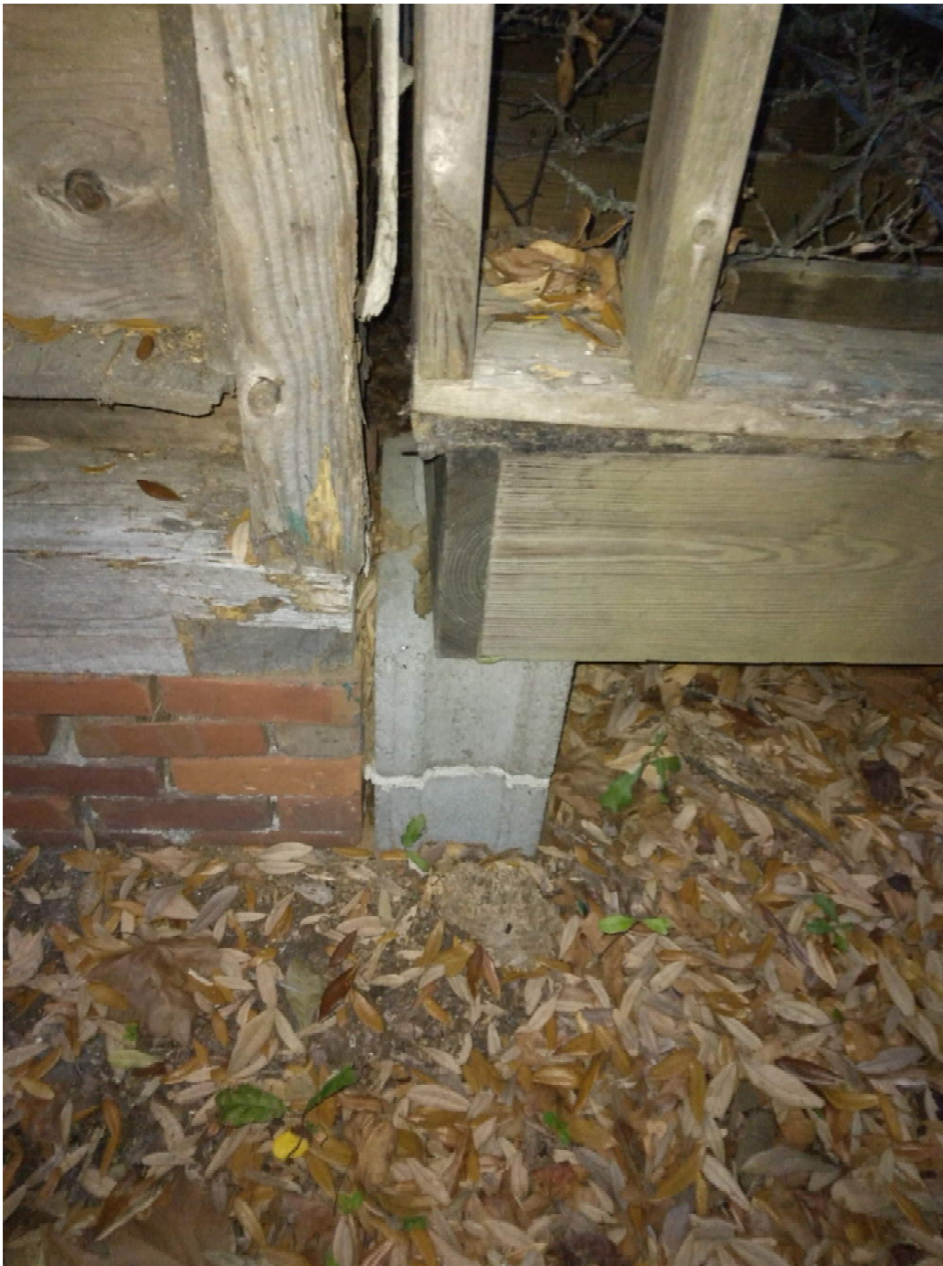
Back Room and North-West Corner connection – No apparent connection of two structures
