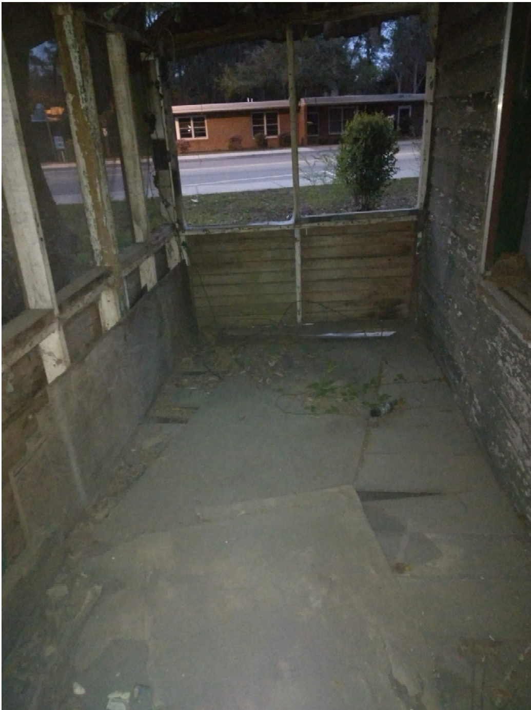
Porch Deck sheathing is rotten and gap between wall and deck
