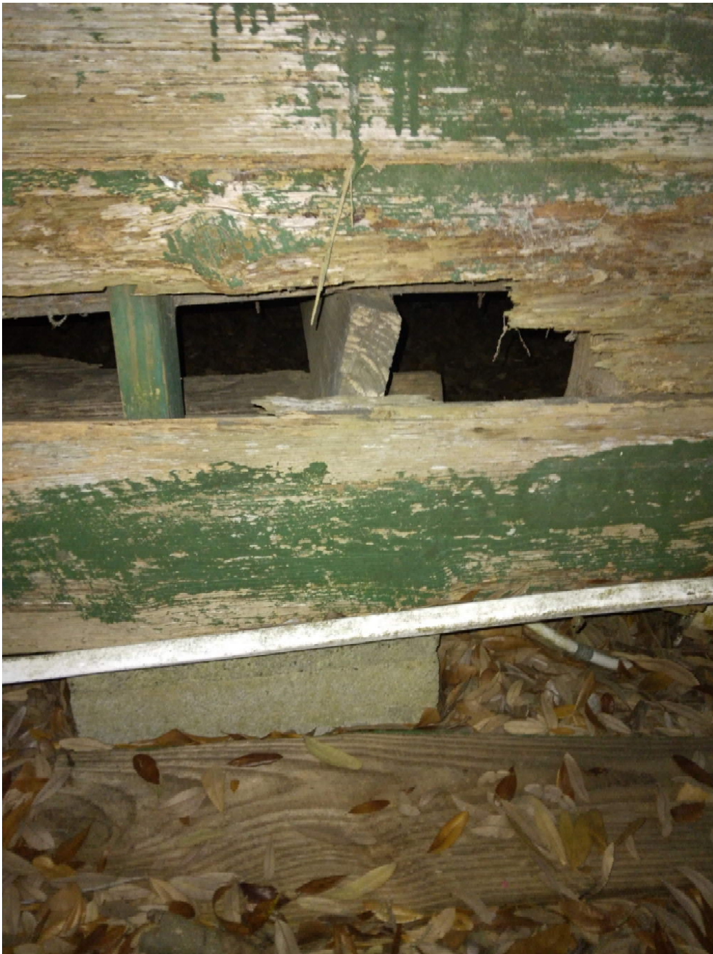
Rotating Floor Joist due to missing band board connection and rotten siding
