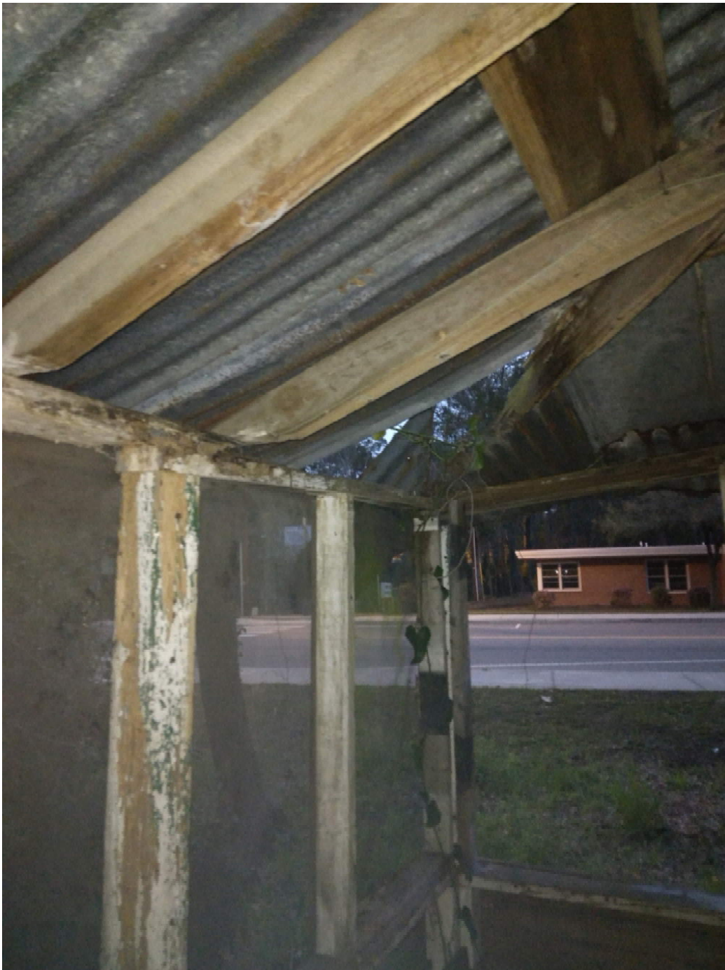
Porch Rotten Top Plate and Roof Rafters
