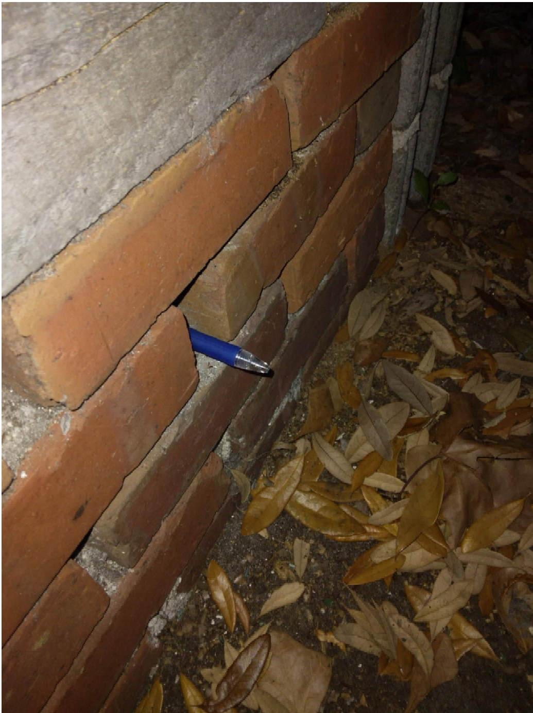
North-West Corner Pier Notice Ball Point Pen in brick joint
