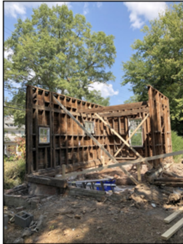
The small accessory structure above was carefully disassembled to allow for its relocation.
