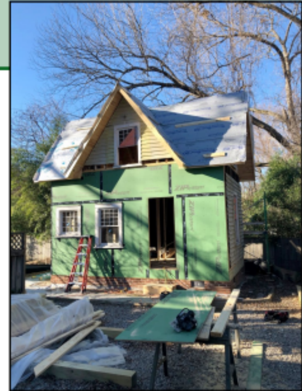
The building was re-assembled on a new site with a brick foundation of similar height to the original foundation.
