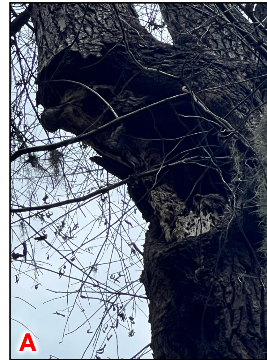
HIC29 - ROTTED TRUNK
