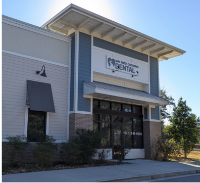
May River Crossing Existing Building
