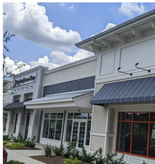
May River Crossing Existing: Recessed & Projecting
