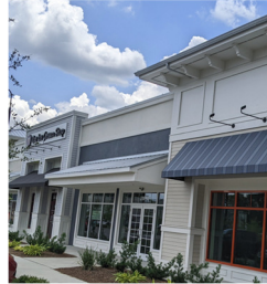
May River Crossing Existing Building – 45% of façade has partial metal roof features - a flat roof is behind the angled metal roof sections
