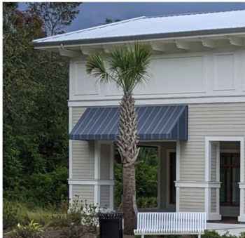
May River Crossing Existing Buildings
