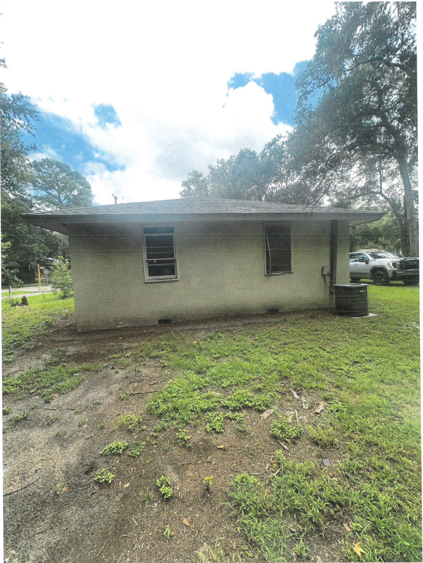
Back - 28 Wharf St
