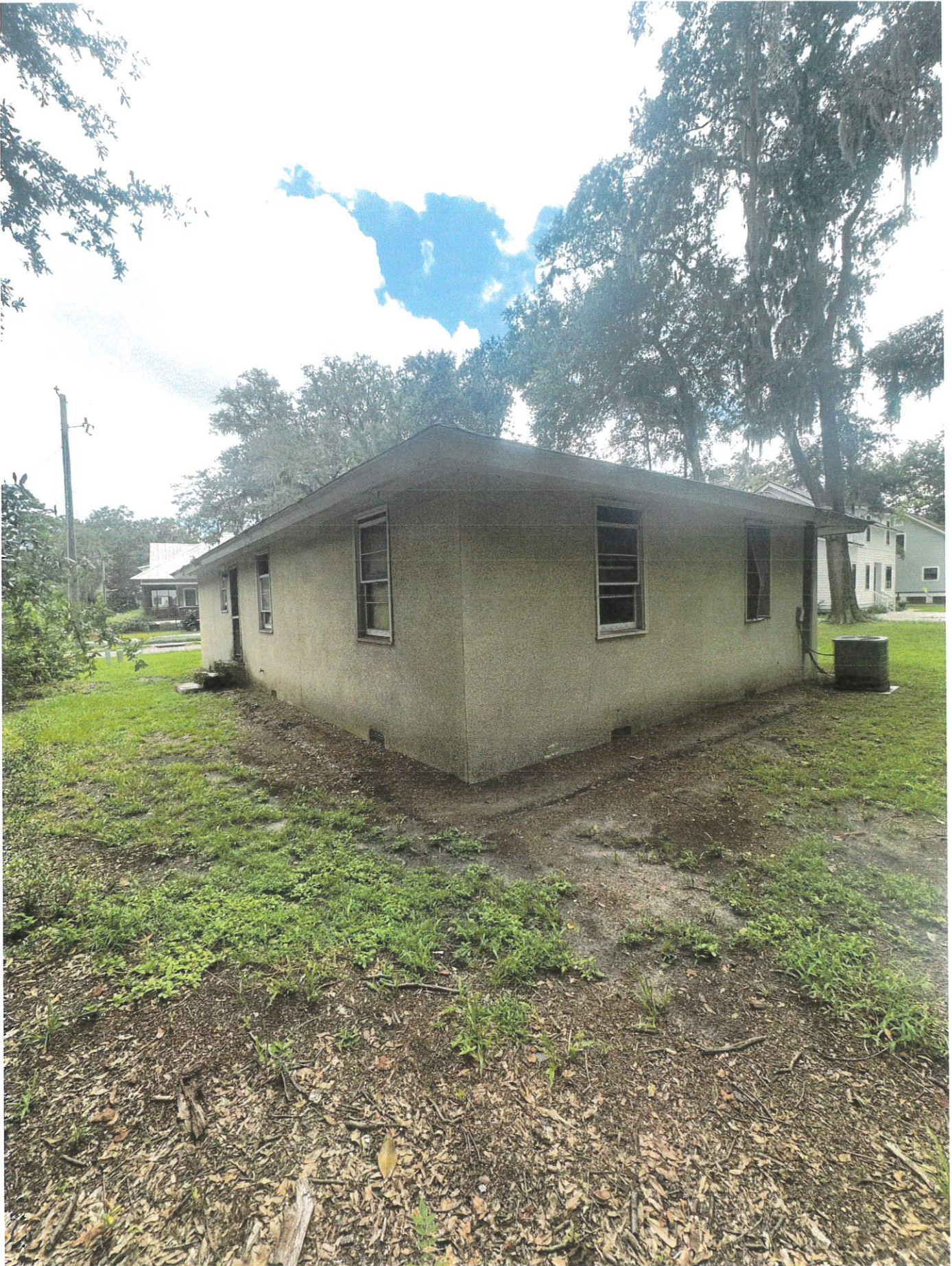
Back Right Corner - 28 wharf st
