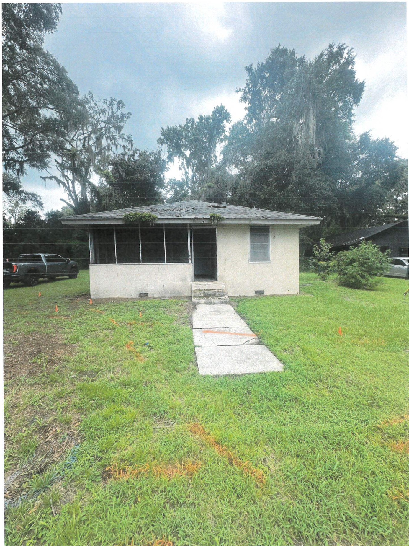
FRONT - 28 Wharf St
