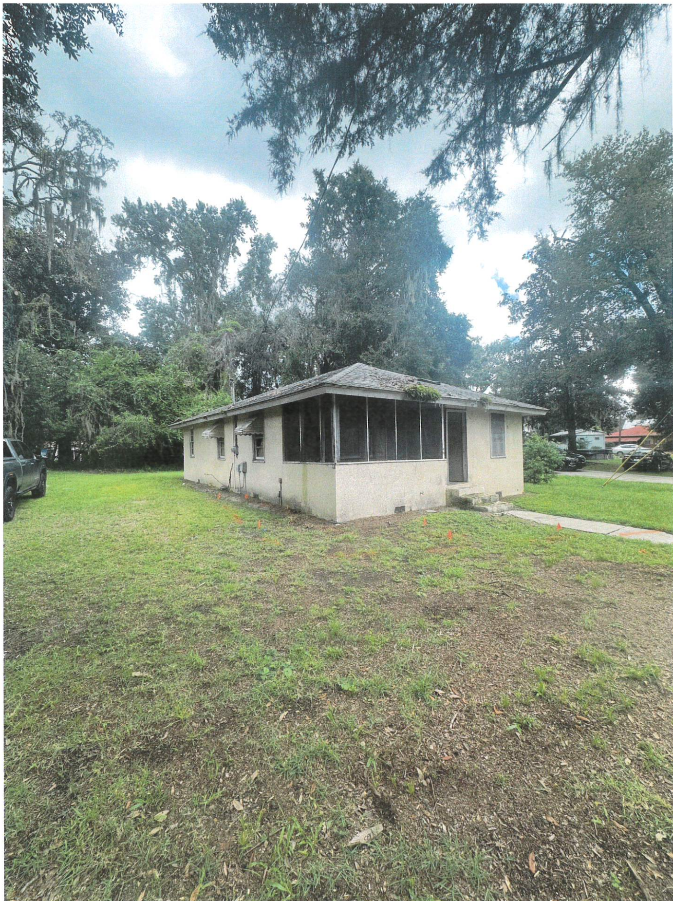
Front Left Corner - 28 Wharf street
