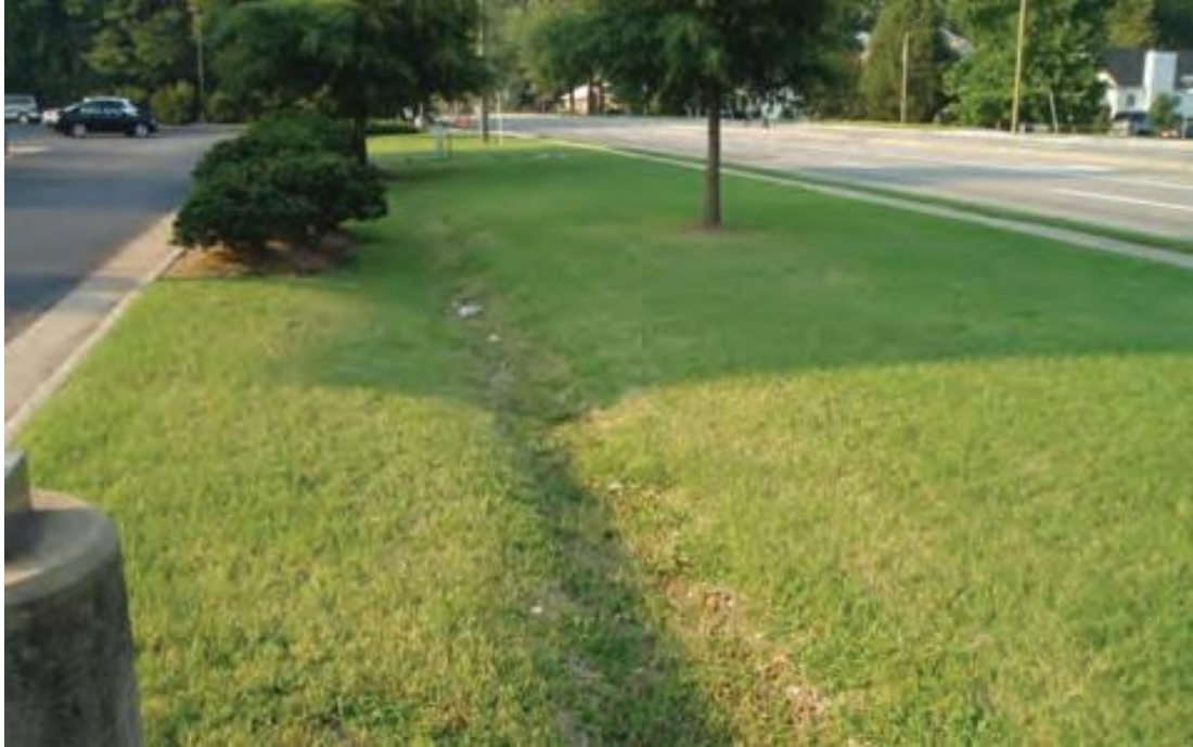
Figure 4.33. Open channel (photo: Center for Watershed Protection, Inc.)
