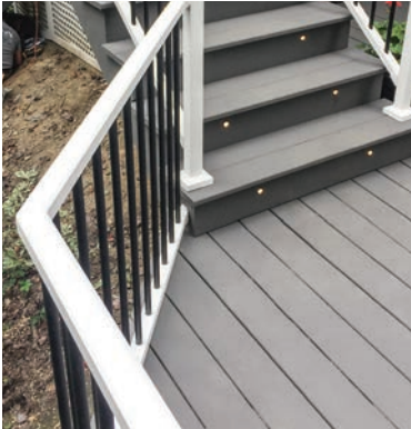
Special Welded Corners
