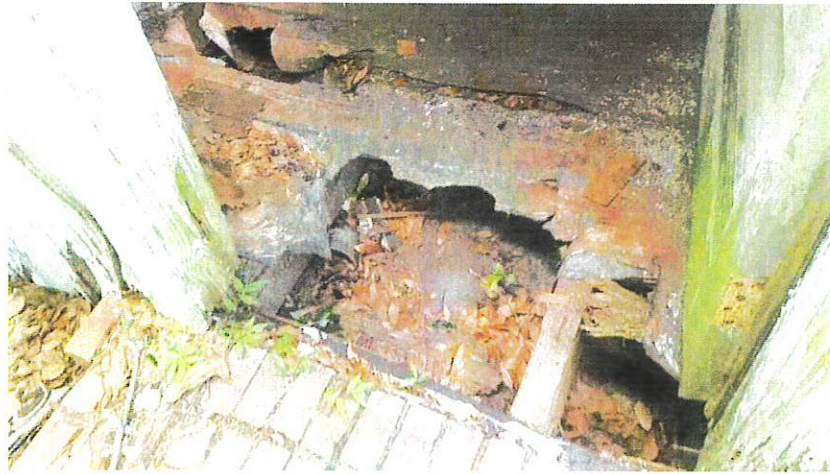
22. Deteriorated floor of BBQ shed
