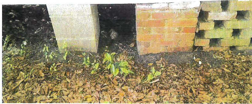
7. Foundation – Rebuilt on left; old on right
