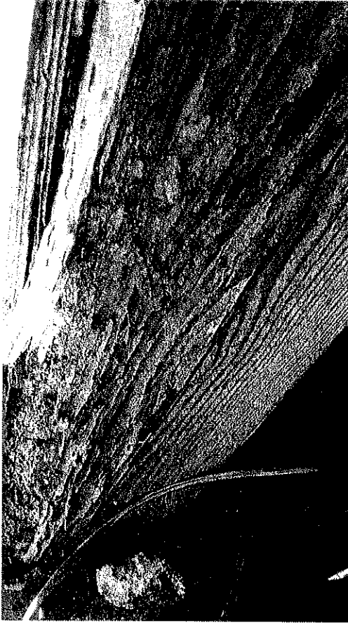
10. Decayed perimeter support beam
