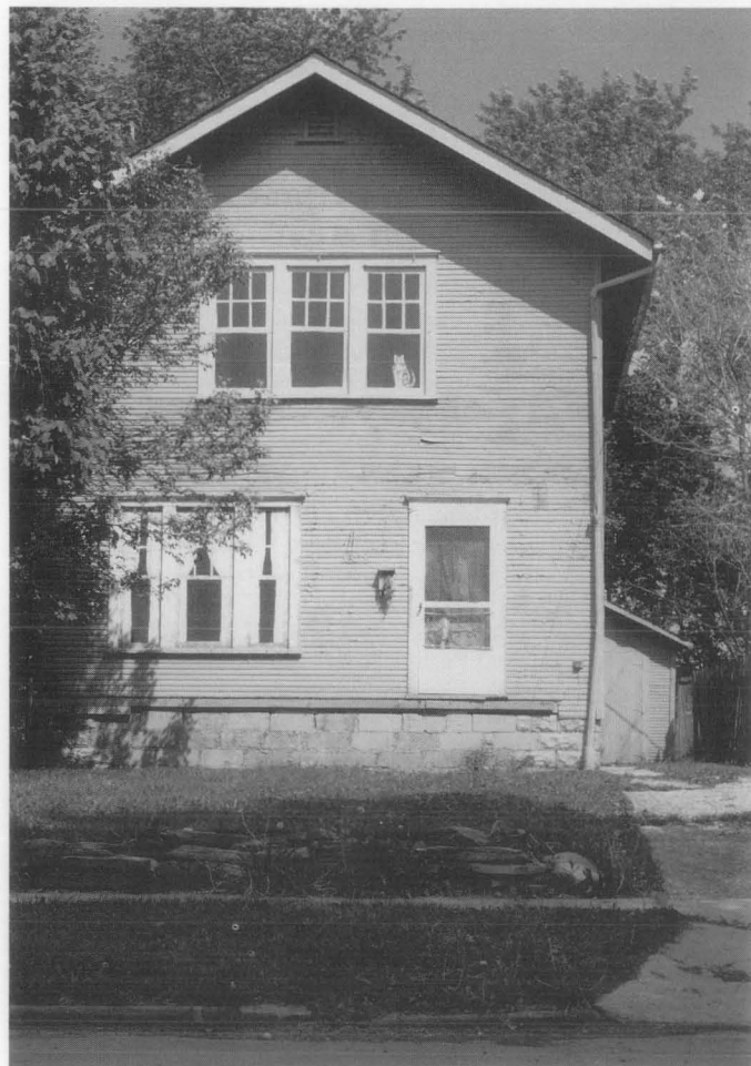
Figure 27. This residential building blends into its neighborhood even though all the windows have been covered over and the front steps are missing. The grounds are maintained and the special attention to decoratively painting the window panels shows that the property is being well cared for until it can be rehabilitated. Photo: Ohio Historical Society.
