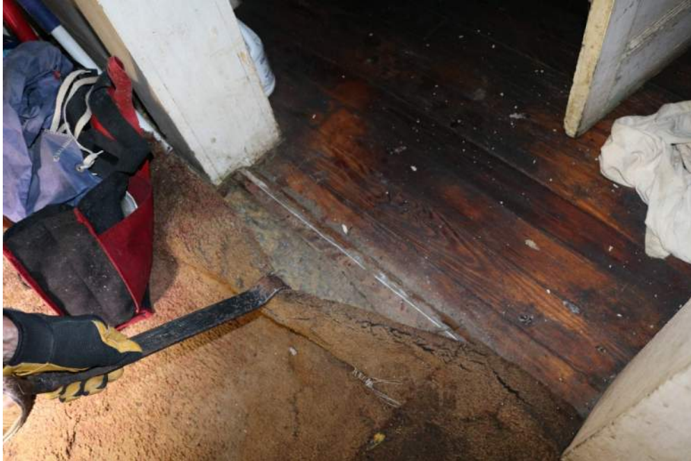
Figure 19: The floor level at the shed-roofed rear portion of the structure, is approximately \frac{1}{2} to \frac{3}{4} of an inch lower than the main floor of the house. This difference could indicate that the rear of the house is later. However, the trim details, the wall covering, and the flooring are the same as the main part of the house. Also, the earliest extant windows are in the rear part of the house. If the rear portion of the house is a latter addition, it appears to have been constructed early in the life of the structure.
