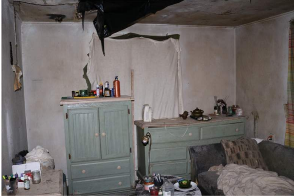
Figure 11: Note the mold covering the walls. The wall and ceiling covering throughout house is a combination of 4 x 8 sheets of plywood with some gypsum drywall. Note the damage to the ceiling. The roof has been leaking for some time, and there is likely damage to the roof framing due to water intrusion.
