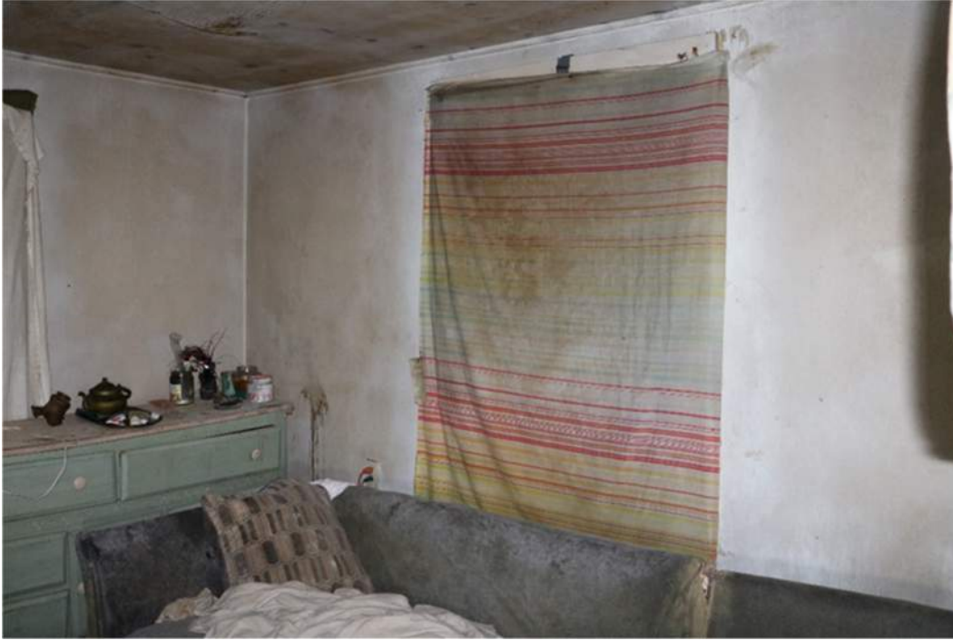
Figure 13: Note the mold covering the walls.
