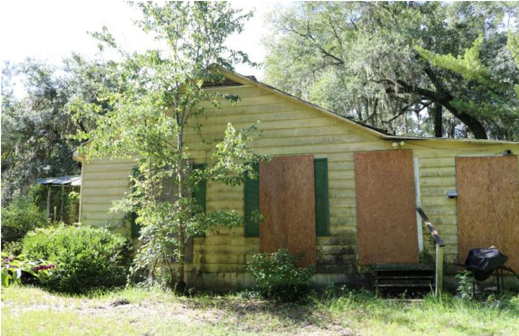
Figure 6: North elevation. All the windows and doors except the front entrance have been boarded up on the exterior.
