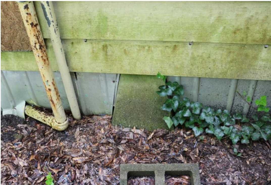
Figure 18: The foundation consists of precast concrete piers. The condition of the footings was not observed, but the Engineer's Report indicated that no adequate footing existed.
