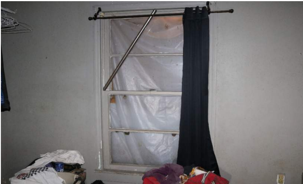
Figure 14: Interior of the house: The window is a later two over two which does not match the light configuration of the windows in the back wall of the shed-roofed rear portion of the structure. The window has aluminum jamb liners and spring balances, which are likely dated to post 1940s. All the windows in the side and front elevations of the structure have aluminum jamb liners with spring balances and are later than the construction date of the house. The two windows in the rear wall of the structure are not balanced and have no jamb liners. These are likely the earliest extant windows.
