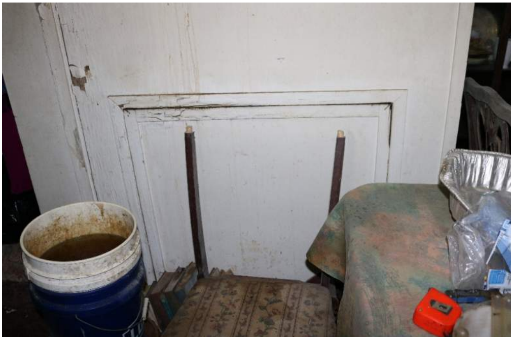
Figure 16: A boxed-out area in the dining room at the location of the chimney. This may cover the location of a removed or infilled fireplace or heat stove.
