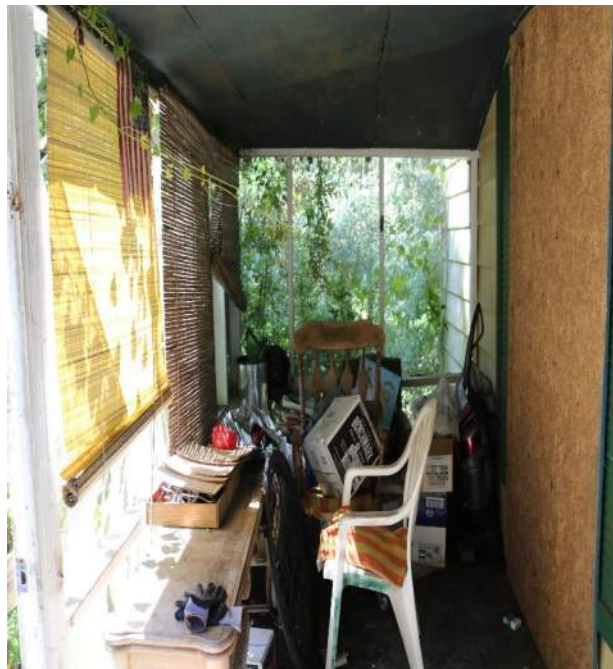
Figure 8: Interior view of the front porch. The framing material of the porch was inspected and determined to be modern and not original to the structure. The porch and the entire interior of the house were filled with abandoned furniture and personal effects. This made the assessment somewhat limited, but did not compromise the final conclusions.
