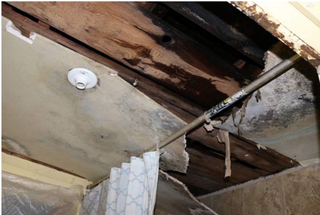
Figure 12: Interior of the house: Note the severely damaged ceiling. The roof has been leaking for some time, and there is likely damage to the roof framing due to water intrusion.
