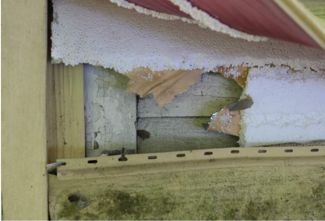
Figure 17: The original siding is in place under the later vinyl siding. The original siding is wood and its condition likely varies from salvageable to completely deteriorated.
