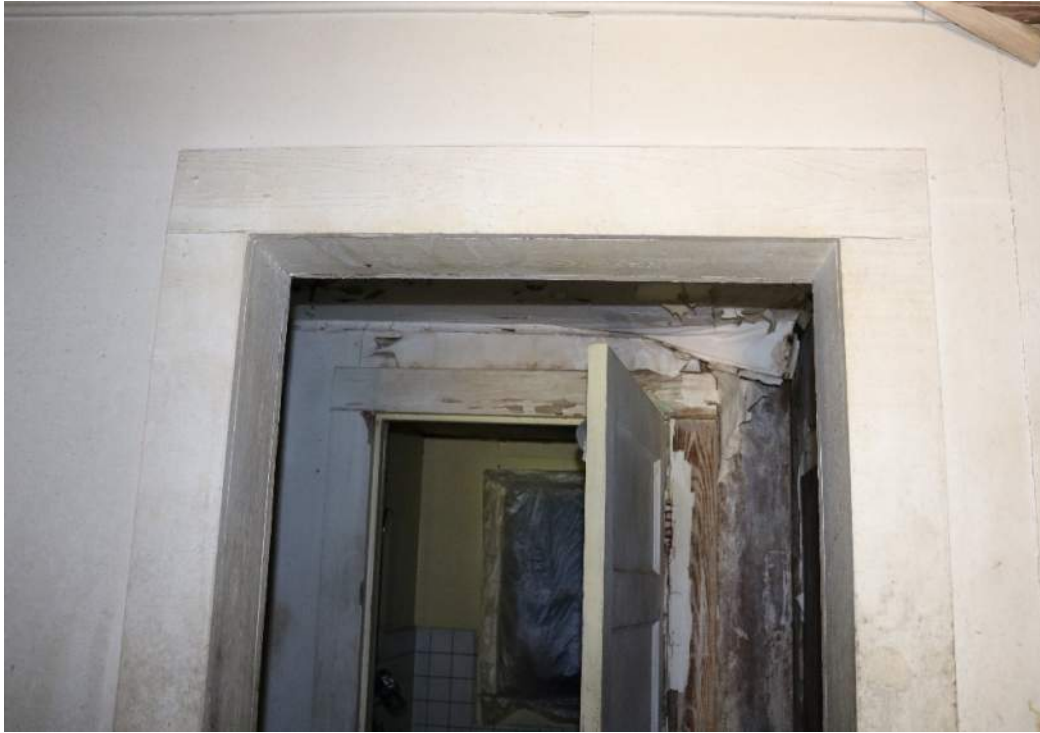
Figure 15: Door trim at the interior of the house. All the door and window trim on the interior of the house is consistent, being S4F 1x6 flat board. The shed-roofed rear portion of the structure maintains this pattern.
