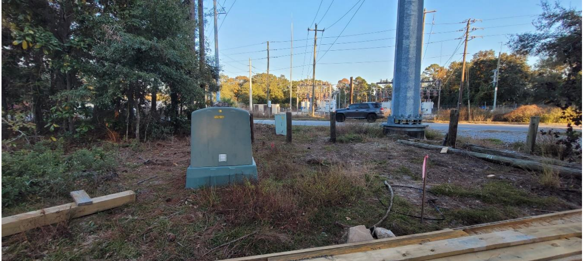
EXISTING DEAD END AT PLUFF MUD LANE
