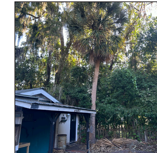
5 LAWTON ST. FACING NORTH EAST CORNER
