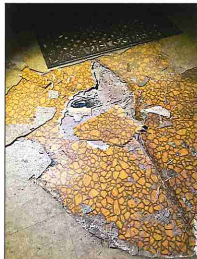
View of living room, bathroom, and kitchen ACM floor covering
